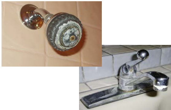
Residents see the affects of salts by deterioration of appliances and fixtures
