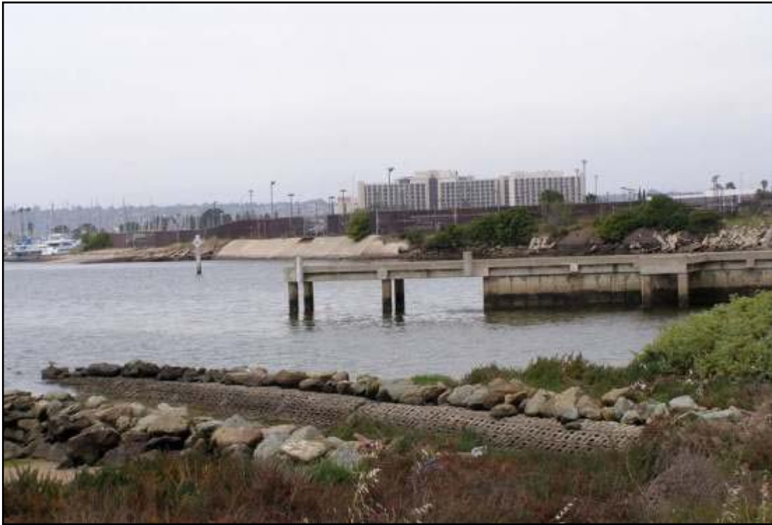
Photo 1: View looking west at the east side of the pier.
