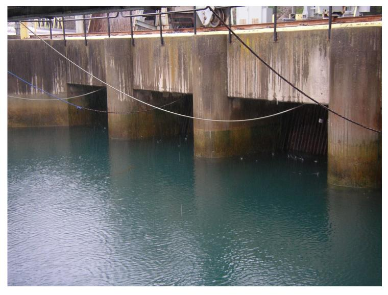
Photo 1: View of the Facility's cooling water intake bar racks and intake structure.
