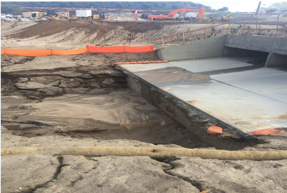
3: Approximately 3-4 feet of sediment eroded and washed downstream of culvert.
