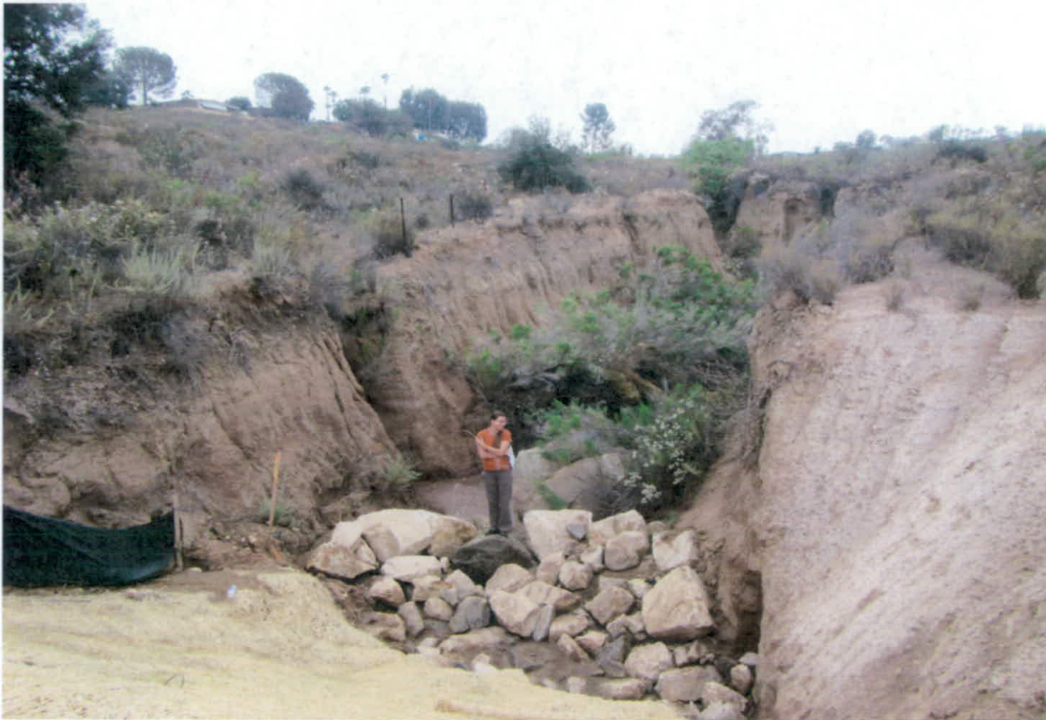
Figure 4. Ephemeral stream in highly eroded canyon, looking west from constructed off-site road knuckle. Photo by Lisa Honma, SDRWQCB, July 1, 2015.
