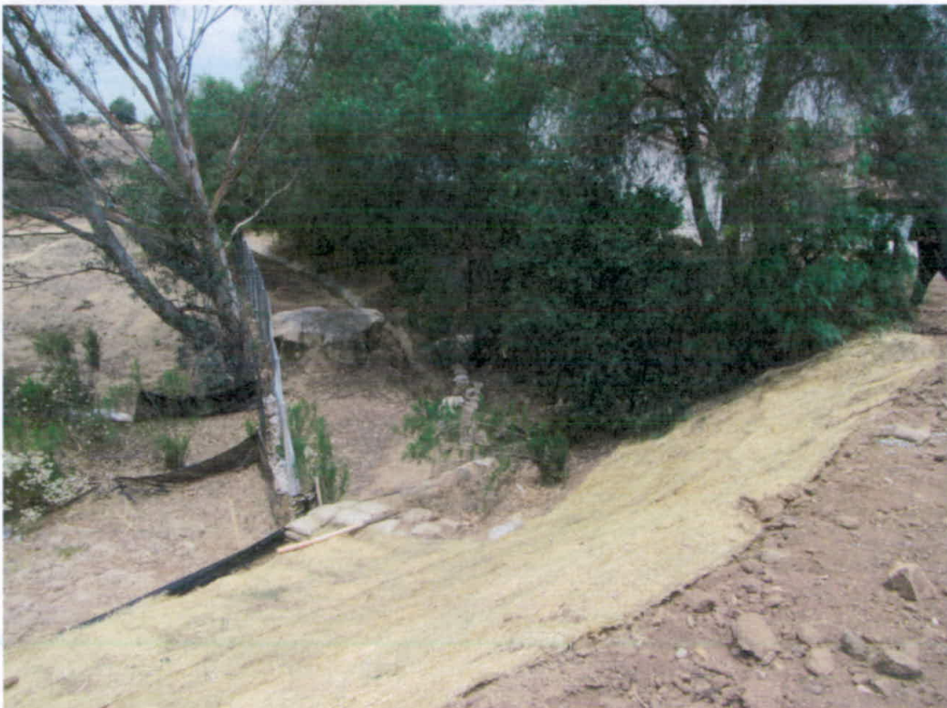
Photo 6: Looking down towards location of storm water inlet 3
