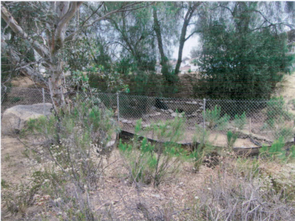
Photo 5: The third storm water inlet structure with construction BMPs in place.
