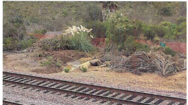
Photo 13 and 14 show discharge from bowl #2 (shown in Photo 8), due to missing sediment or erosion controls.
