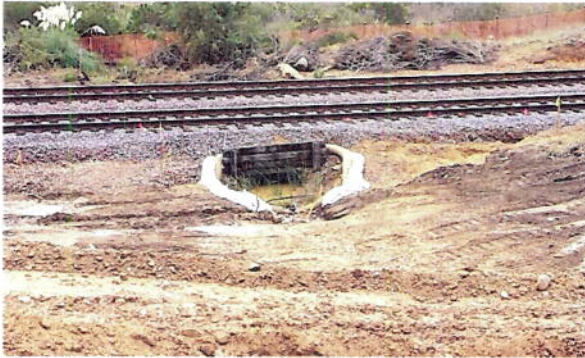
Photo 13 and 14 show discharge from bowl #2 (shown in Photo 8), due to missing sediment or erosion controls.
