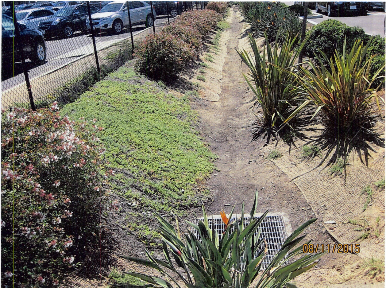
Photo 6(g): Larger bioswale at southerly boundary of auto dealership. Floor of the bioswale channel is hard packed earth which showed no indication that it had ever been previously planted with vegetation. Based on input from City inspector in 2015, the owner added burlap matting and planted ornamental vegetation on the sides of the bioswale (apparent miscommunication between owner and inspector).
