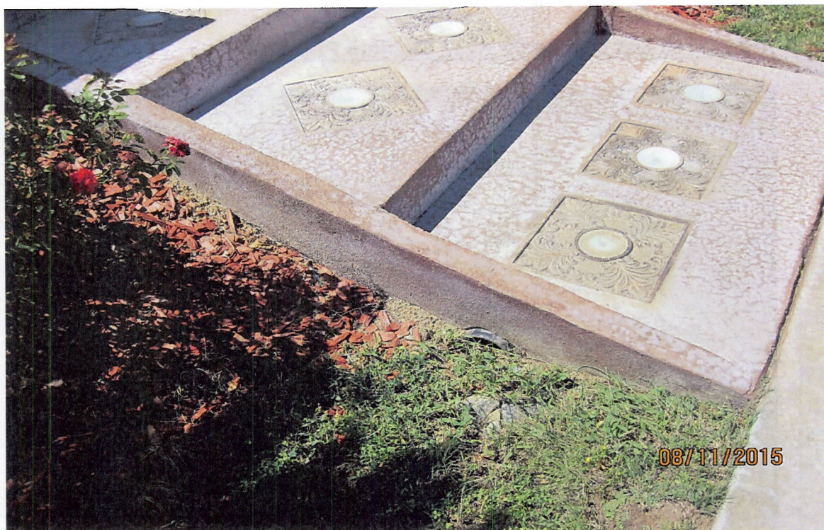
Photo 3(i): Stairs constructed in the middle of bioswale. Flow through pipe is buried 2/3 of the way below swale.
