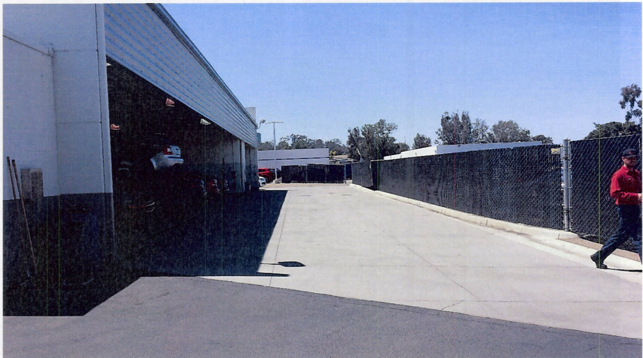
Photo 6(b): Back service bay that feeds into smaller swale in back of dealership. Questions remain if car storage lot to the right of the fence is part of dealership and needs treatment.
