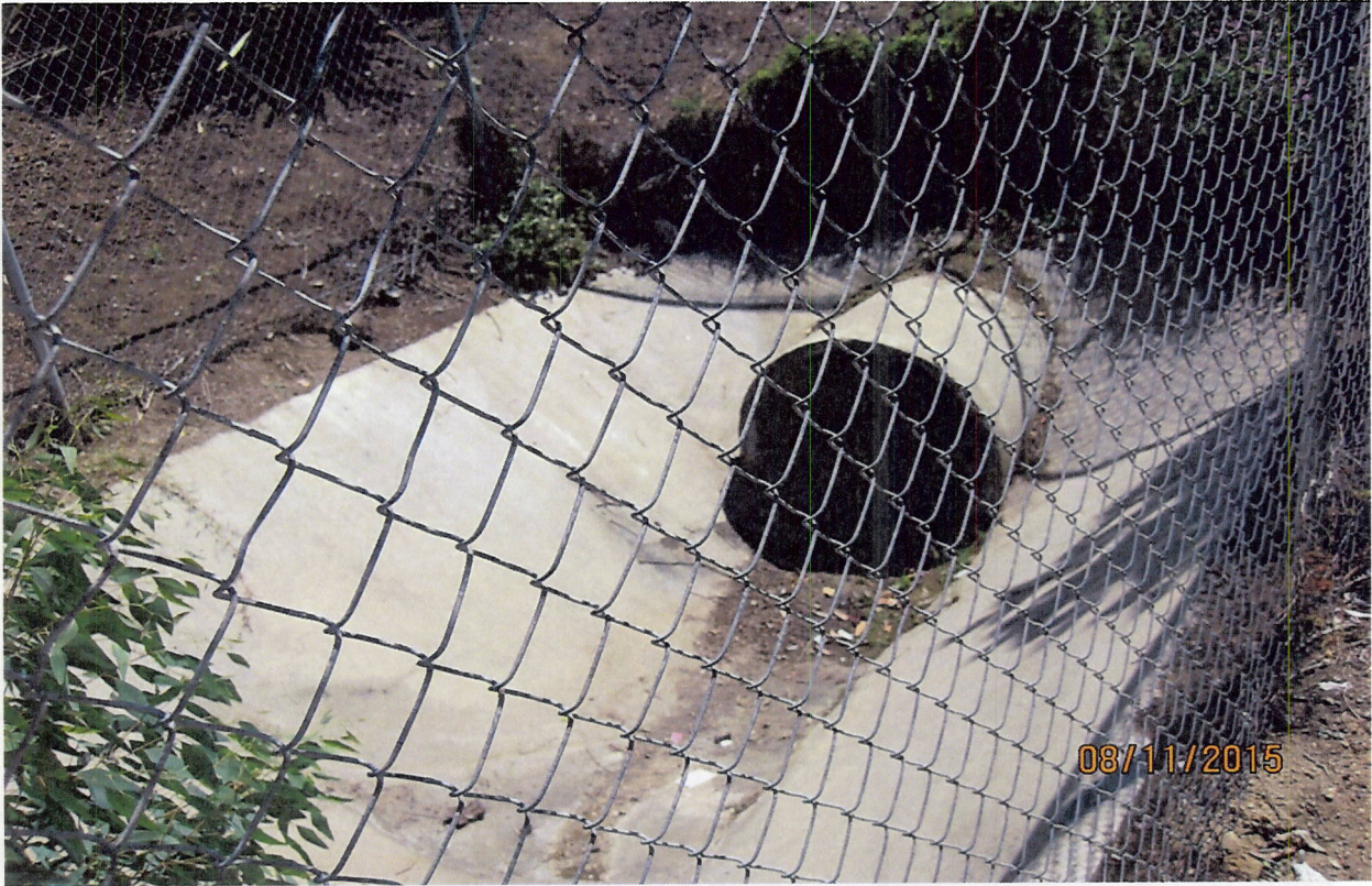
Photo 6(e): Small swale discharges directly into City of Escondido MS4 system.
