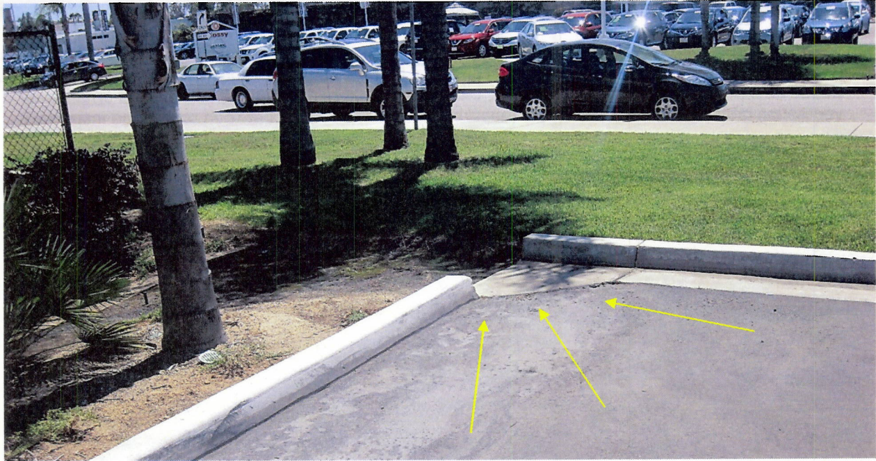
Photo 6(f): Single curb cut inlet to larger bioswale from front of dealership parking lot.
