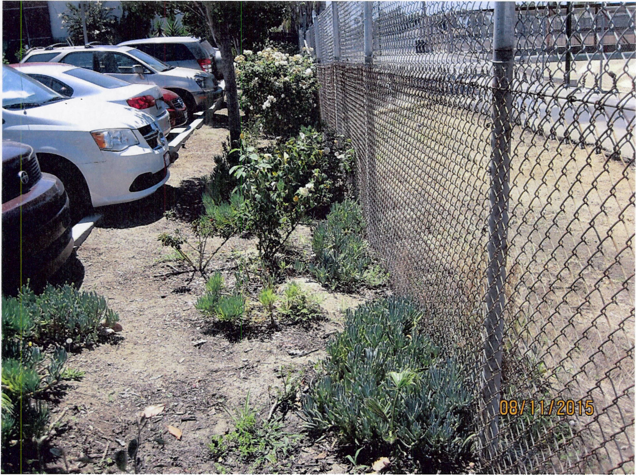
Photo 5(c): Area of parking lot on site that appears to be the actual location of the bioswale per the original plans. This area could be re-graded and planted with vegetation to better serve as a treatment control BMP for the site. As it exists now, the area slopes downward towards the fence and the offsite dirt area beyond the property boundary.
