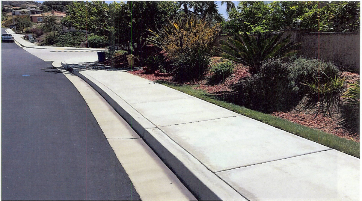
Photo 3(j): Landscaping with ornamental bark covers the upper side of the swale, reducing ability to treat stormwater.
