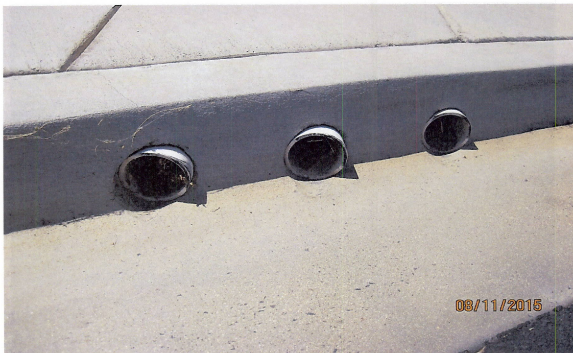
Photo 3(d): Inlet pipes clogged with sediment. Flow is not able to get into swale, backs up and some sediment is deposited.
