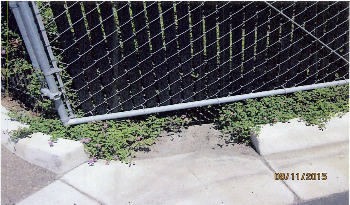
Photo 6(c): Curb cut that serves as the inlet to the smaller swale in back of dealership.
