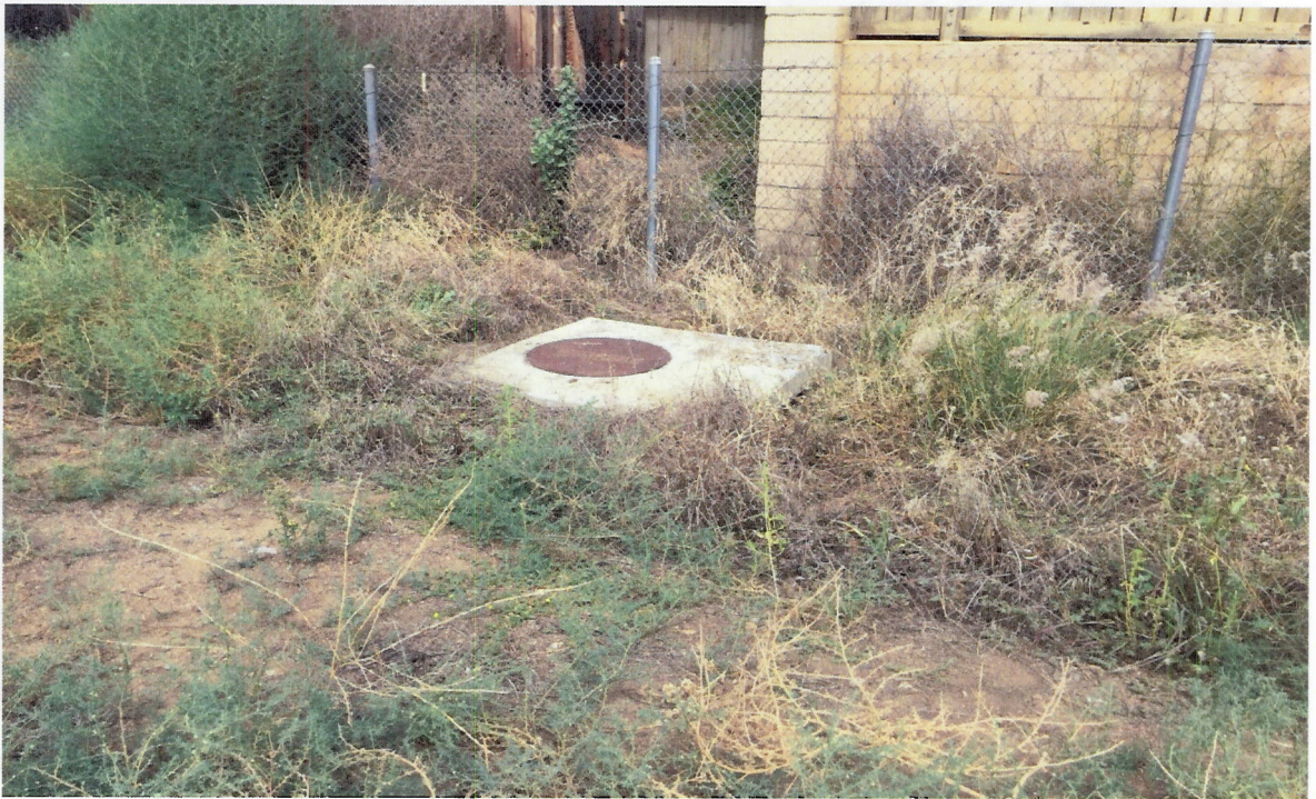
Photo 2(d): Inlet structure at the terminus of the Bioswale.
