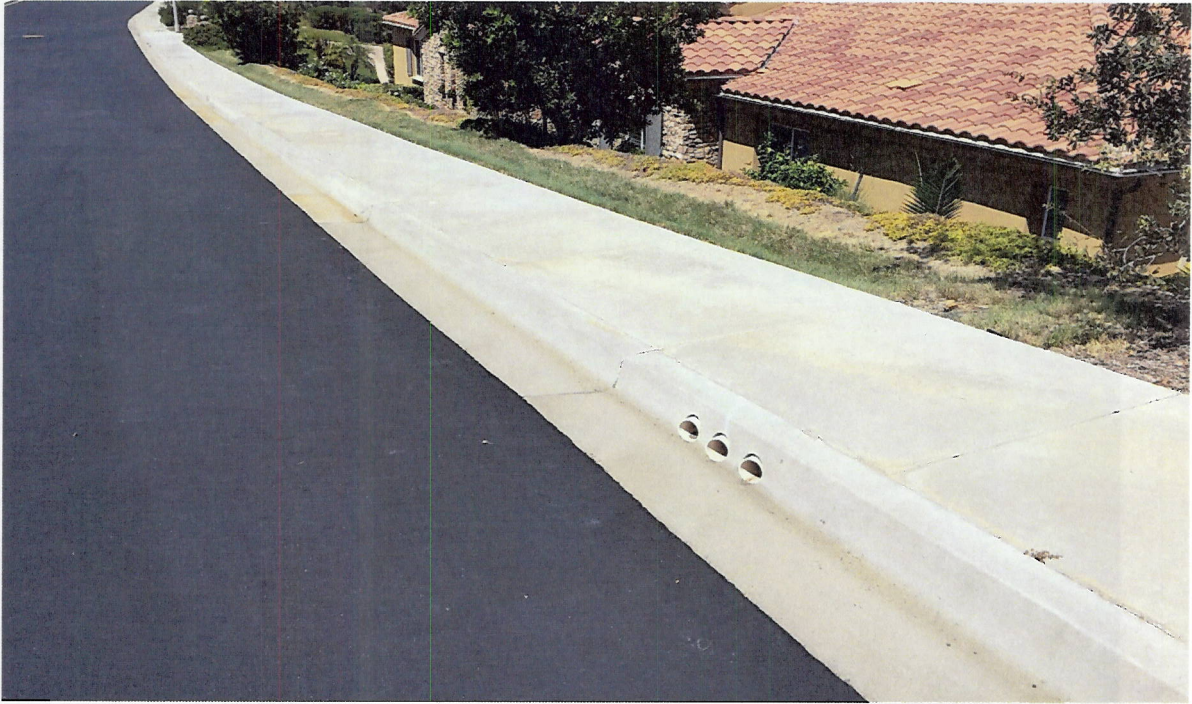
Photo 3(b): Typical bioswale set up with three inlet pipes and vegetated swale running along street.
