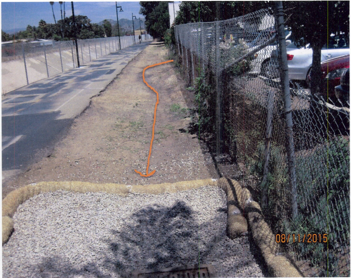
Photo 5(b): Past location of bioswale within City right away adjacent to Escondido Creek. Orange line shows the approximate flow path of stormwater exiting parking lot through single curb cut. Flow would tend to pass at a right angle through lightly vegetated area at the top of arrow, flow through unvegetated area and eventually enter protected storm drain inlet at bottom of picture. Stormwater runoff would receive little or no treatment.
