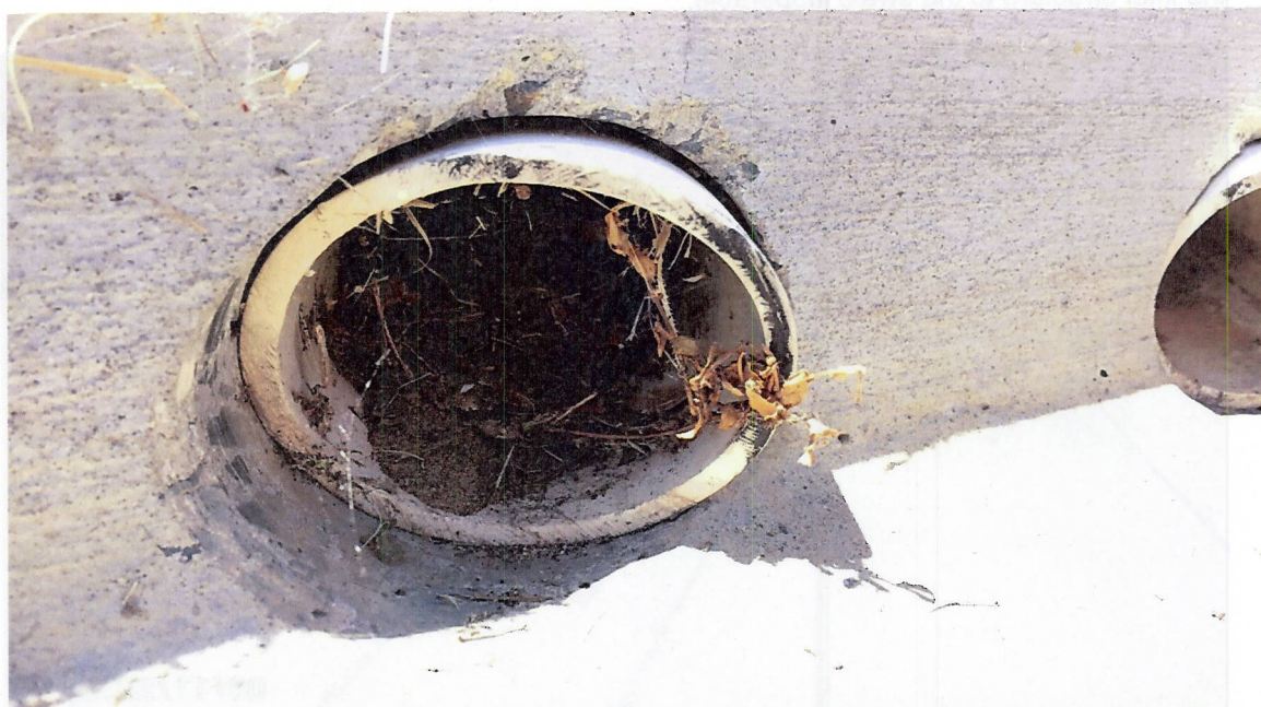
Photo 3(d): Inlet pipes clogged with sediment. Flow is not able to get into swale, backs up and some sediment is deposited.
