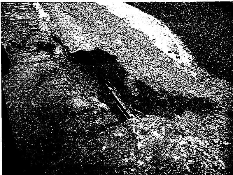
688. A closer look at one of the erosion gullies in photo 686 shows exposed irrigation pipes.
