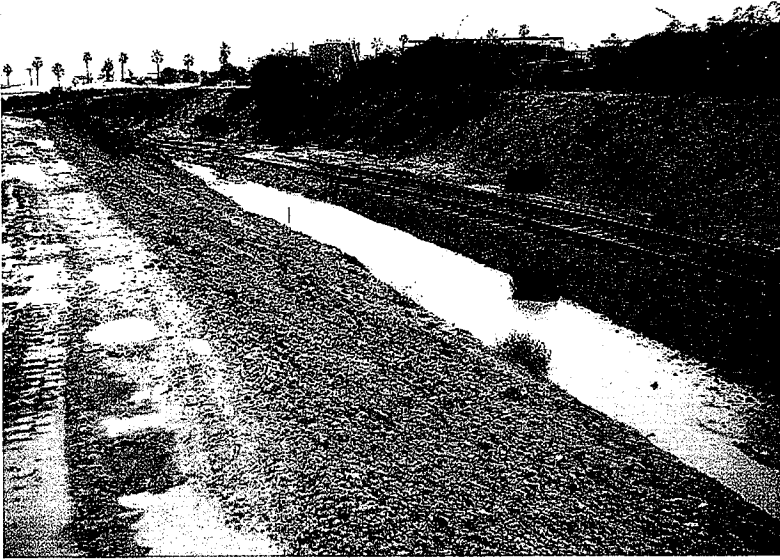
689. This photo shows where construction ended. The far slope is vegetated and the rail ballast rock is a different color. The slopes have no erosion or sediment controls.
