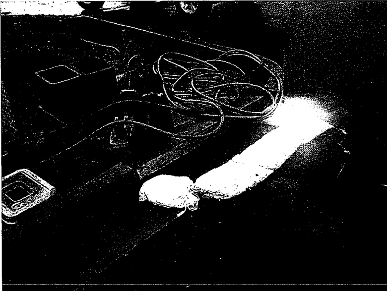
699. Storm drain inlet has been protected. This was in response to deficiencies noted on Tuesday, November 27, 2007.
