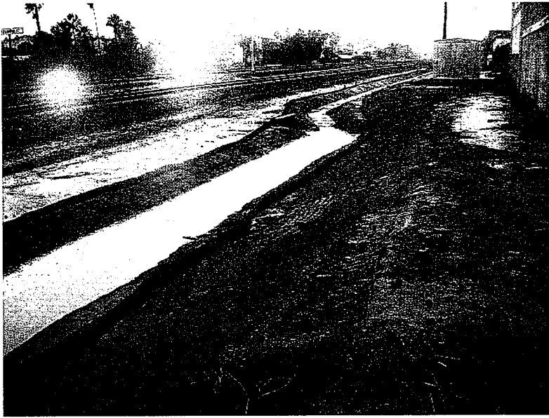
669. Unlined dirt storm drain channel full of sediment laden water.
