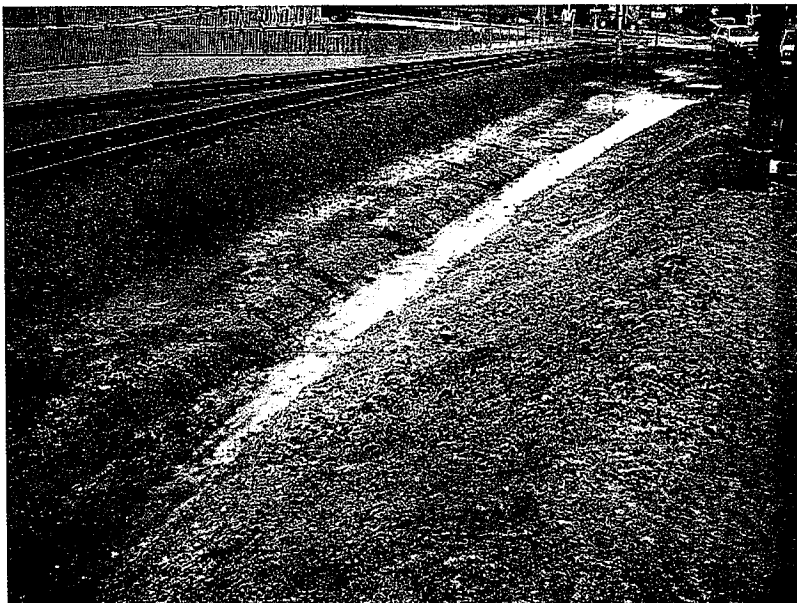
691. The same dirt channel in the previous photo leads to the far storm drain inlet.
