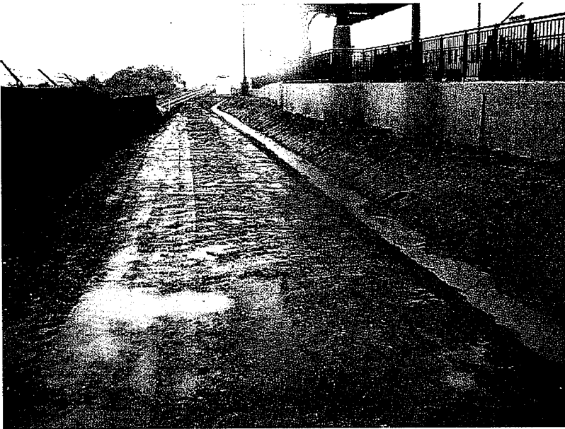
756. Unlined dirt channel leading to the inlet in photo 754 is running with sediment laden water.
