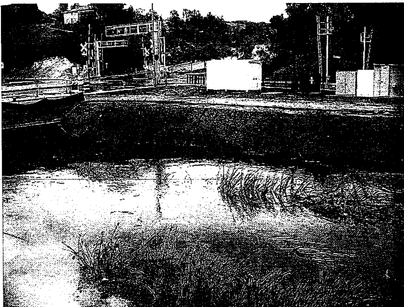
707. The bank of Loma Alta Creek has been sprayed. This was in response to deficiencies noted on Tuesday, November 27, 2007. The application appeared light.
