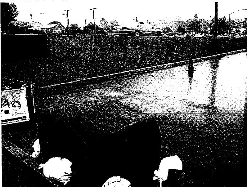
732. Construction materials are covered. The slope is sprayed with erosion control.
