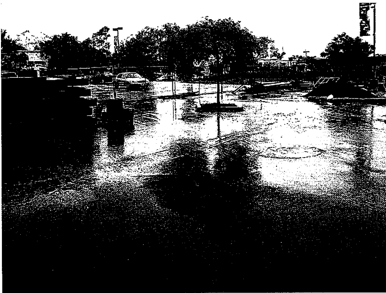
715. Sediment has not been swept up prior to rainfall on a parking lot used as a staging area for construction.
