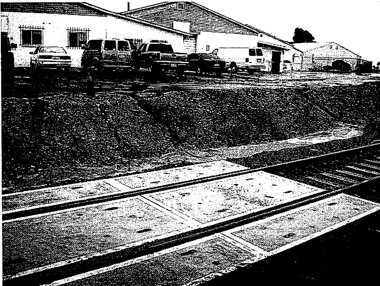
686. A slope with no erosion or sediment controls has large gullies.
