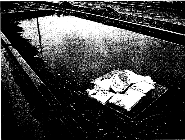
700. Storm drain inlet has been protected. This was in response to deficiencies noted on Tuesday, November 27, 2007.
