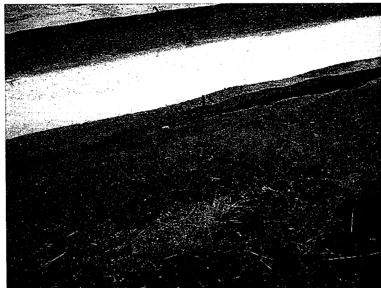
671. Slope erosion from offsite runoff not being addressed.
