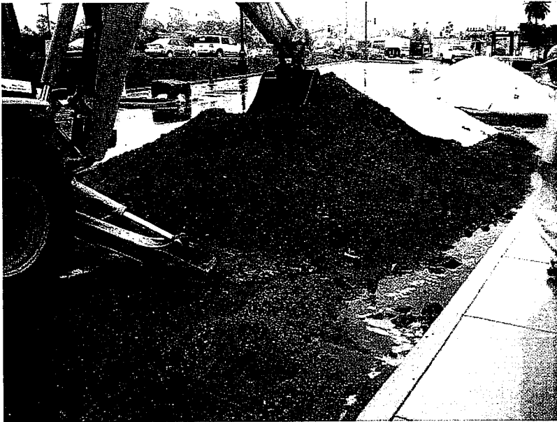
730. Soil stockpile is not covered or protected from storm water.
