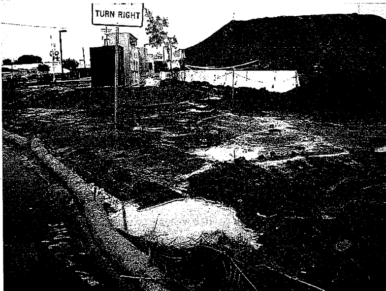
765. The source of the sediment laden water discharging in photo 764.
