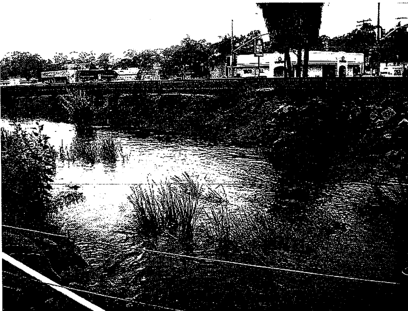
698. The far slope has been sprayed with erosion control. This was subsequent to deficiencies noted on Tuesday Nov. 27, 2007.
