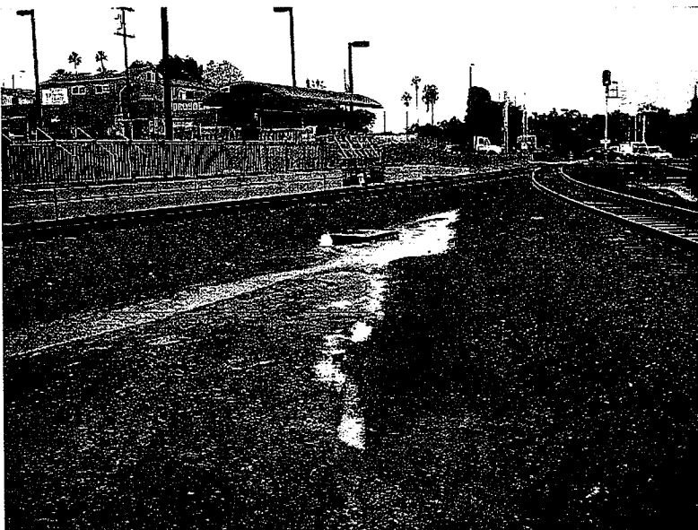
684. A storm drain inlet without adequate protection is receiving a sediment laden water discharge.
