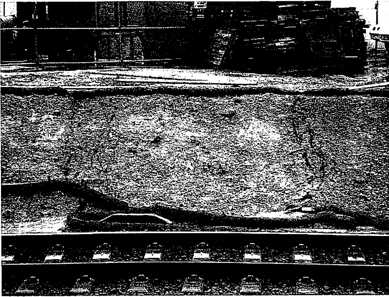
681. Erosion gullies are present on a slope.
