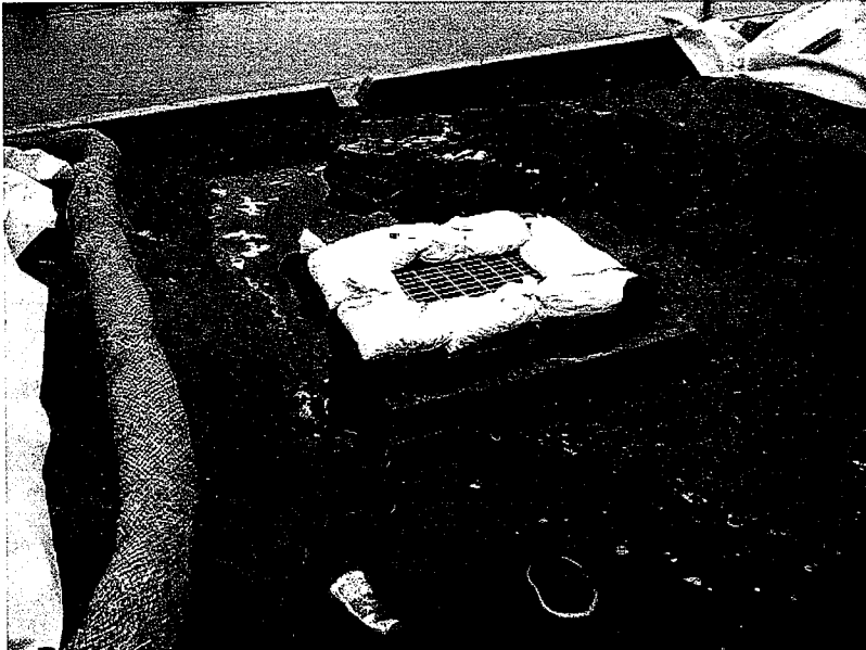
731. Storm drain inlet is protected.
