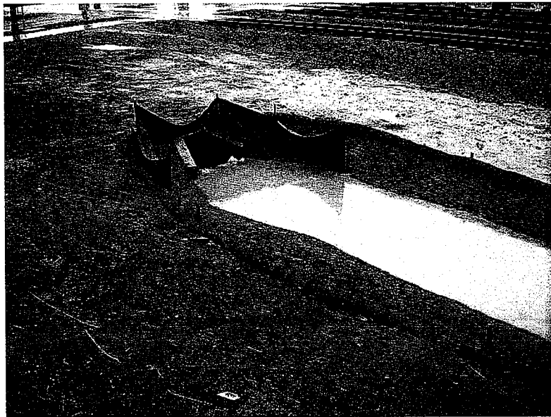
670. The sediment laden water pours into this inlet with inadequate sediment control protection. This deficiency was also noted on Tuesday, November 27, 2007.
