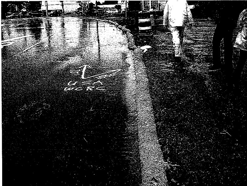
Photos 764 to 772 were taken at Nordahl Road Station in San Marcos.
