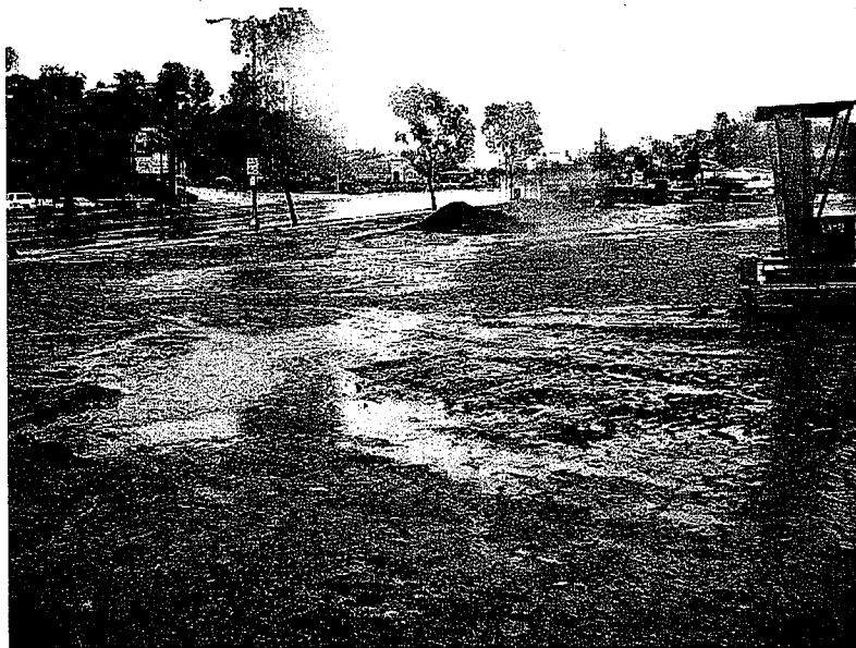
745. Sediment laden water flowing across the construction storage yard to the inlet in photo 746.
