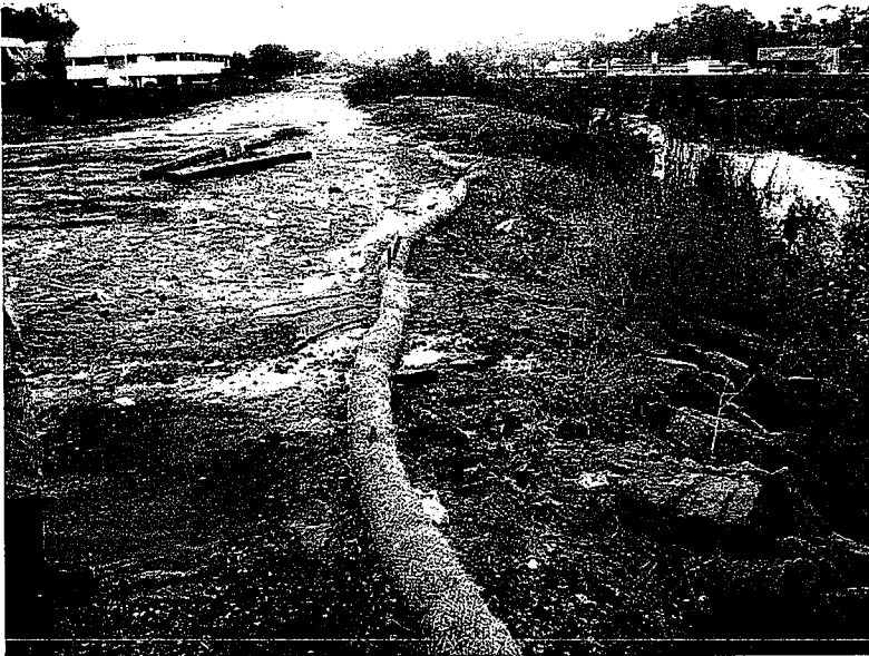
695. Fiber roll along the top of the bank to Loma Alta Creek has not been trenched in.
