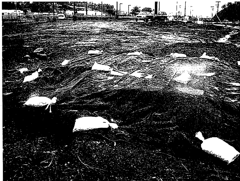
694. Remnants of an asphalt cold mix stockpile have been covered with plastic. This was in response to a deficiency noted on Tuesday, November 27, 2007.
