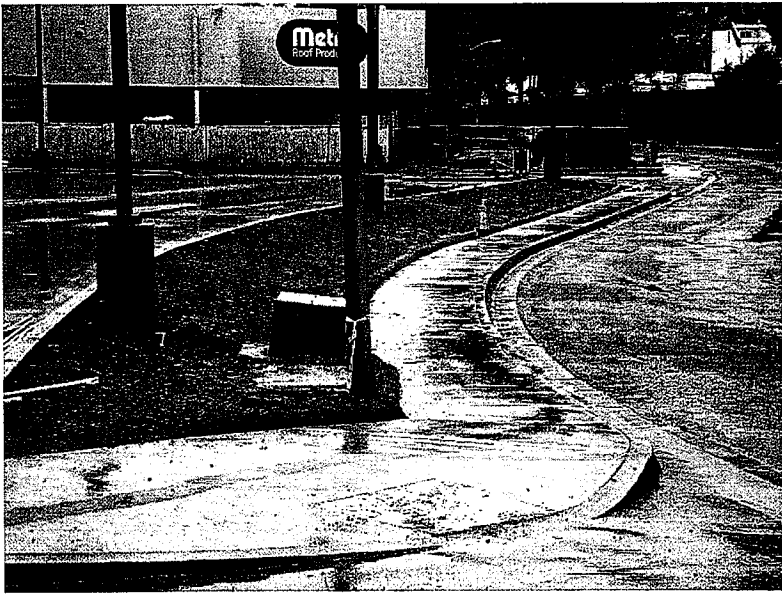
705. Fiber roll has been implemented behind the sidewalk. This was in response to deficiencies noted on November 27, 2007.
