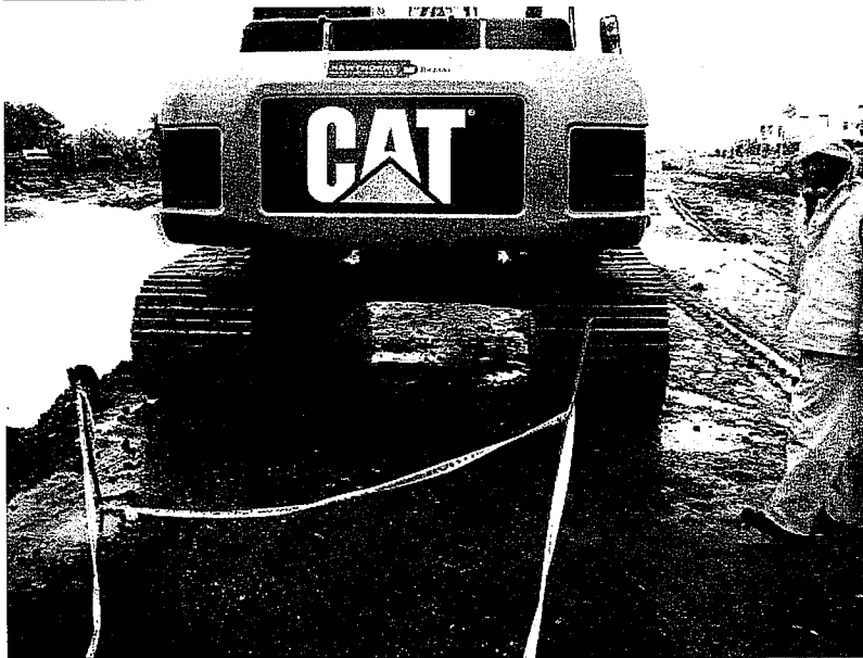
770. Construction equipment is stored without drip pans. No drip pans were present under any construction equipment. This is just one example.
