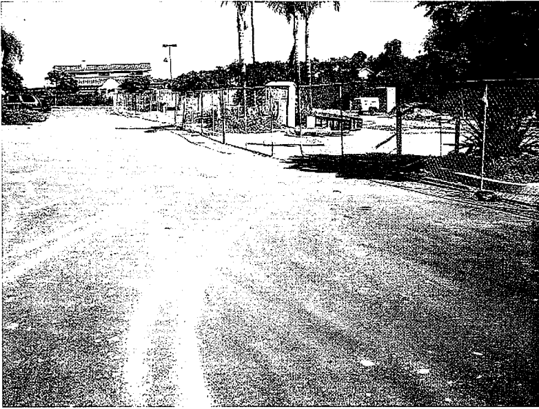
37. Sediment tracking from the College Station construction onto the paved parking lot of the shopping center. Photo looking east.
