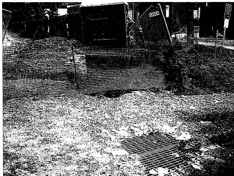
24. Another view of the inlet in photo 23 shows the proximity of a portable toilet and silt fencing that has been partially removed. Photo looking north.
