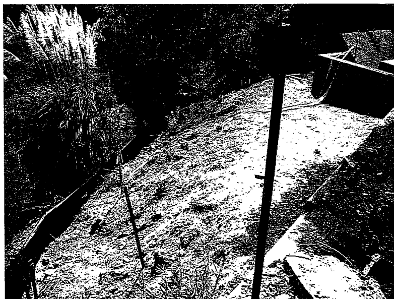
39. Slope next to Loma Alta Creek pedestrian bridge abutment is without erosion controls. Photo looking west.
