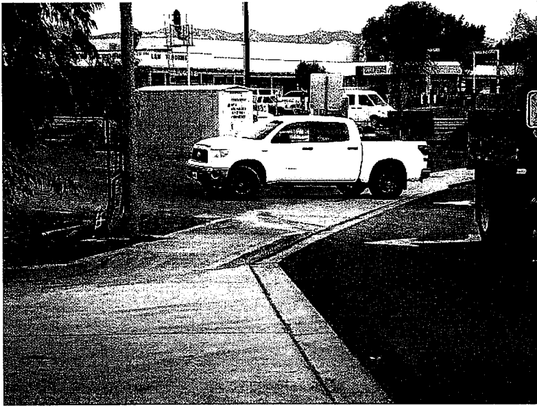
10. Construction site exit has no BMPs to prevent sediment tracking. Tracking is observed onto the adjacent paved public street, North Citracado Parkway. Photo looking north.
