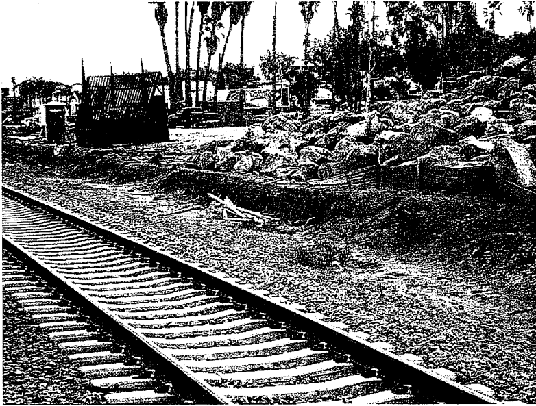
13. Silt fence south of the tracks is torn down and unmaintained. Photo looking south east.
