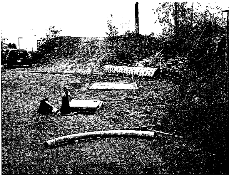
17. Construction trash is not protected with BMPs from storm water. Photo looking east.
