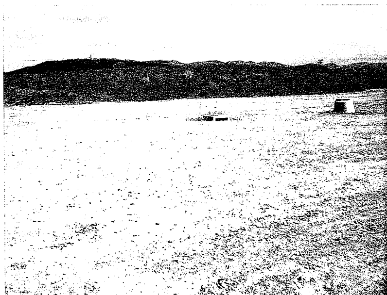
21. A large area of bare soil is without soil stabilization. A storm drain inlet sits in the middle of this bare area.
