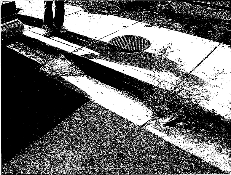
7. Storm drain inlet along the south side of Washington Avenue is without adequate storm drain inlet protection. The existing BMP has not been maintained. Photo looking south.
