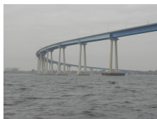
San Diego Bay bridge
