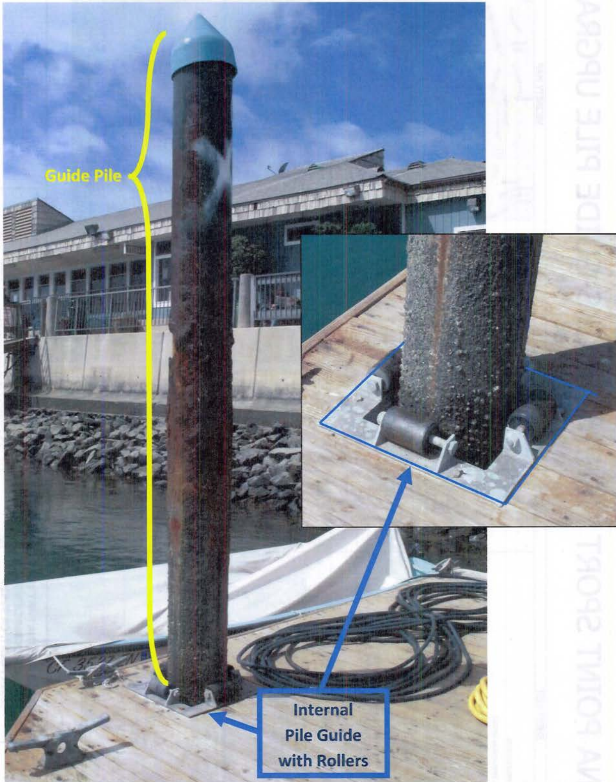
Figure 3: Guide Pile and a Pile Guide on Dock 1
