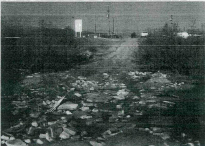
View of on-site drainage and illegal dumping activities.
