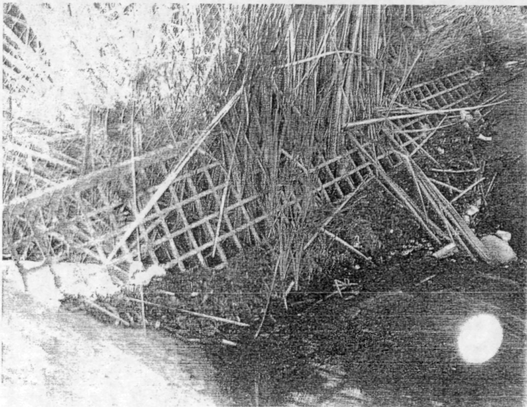
Figure 4 - Trash rack at the west end of channel showing presence of immature cattails.
