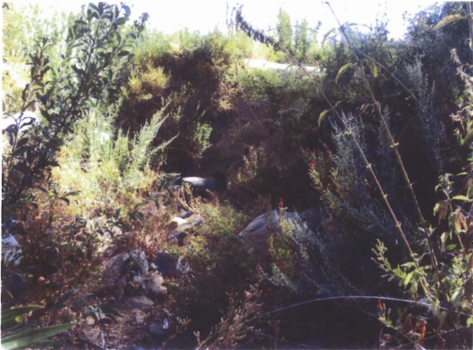
Cold Stream channel upstream of the SR-79 Culvert inlet.
