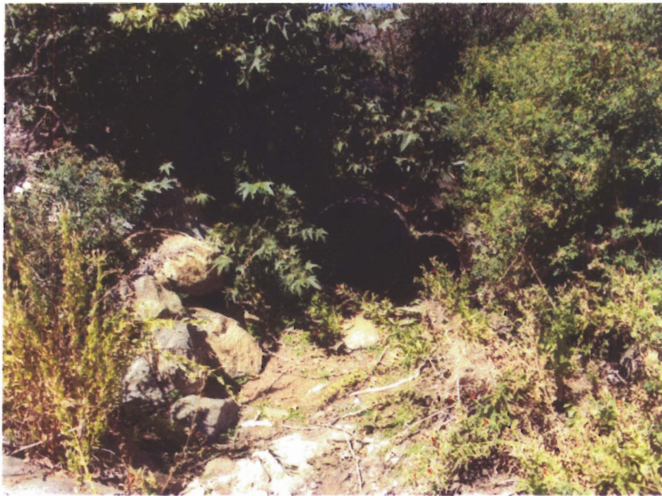
Cold Stream channel downstream of the SR-79 Culvert outlet.
