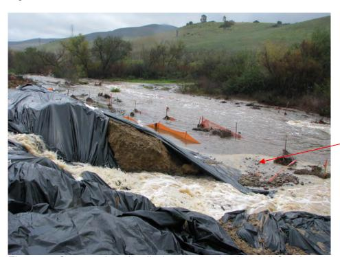
Figure 8. Construction site discharge entering Lusardi Creek
