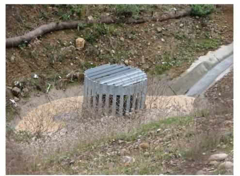
Riser pipe is wrapped with filter fabric. Note turbid water surrounding pipe entering via concrete swale.
