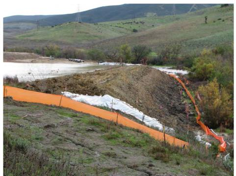
Figure 4. Berm used to detain storm water
