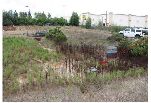
Figure 2. Desilting basin inside project boundaries
