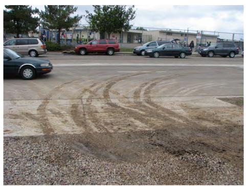
Note sediment on street. Gravel BMP in poor condition and in need of maintenance.
