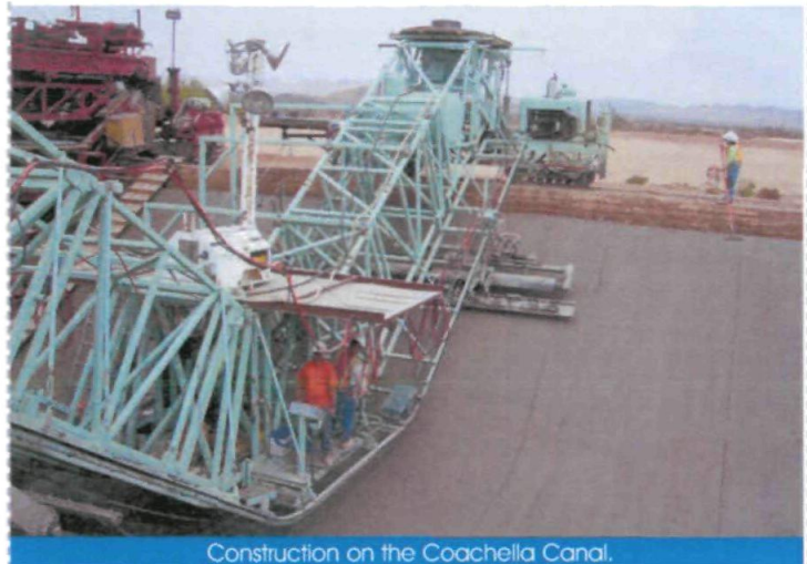
Construction on the Coachella Canal.
