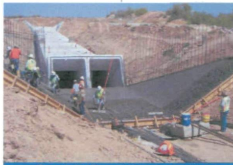
Coachella Canal lining construction
