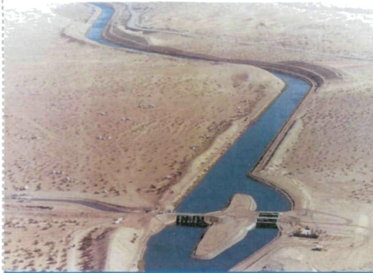
Construction on the All-American Canal lining project began in 2007.
