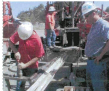
Drillers work at the Mission Basin Brackish Groundwater Desalting site.
