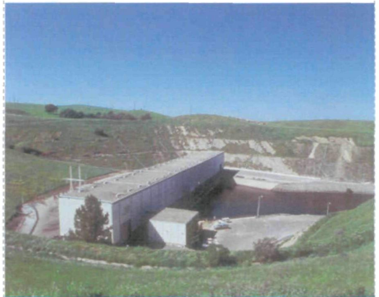
The SWP's Banks Pumping Plant lifts water to the California Aqueduct.
