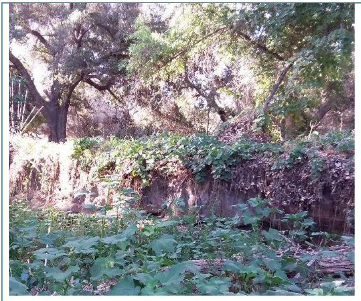
Figure 14 Example of significant stream bank mass wasting
