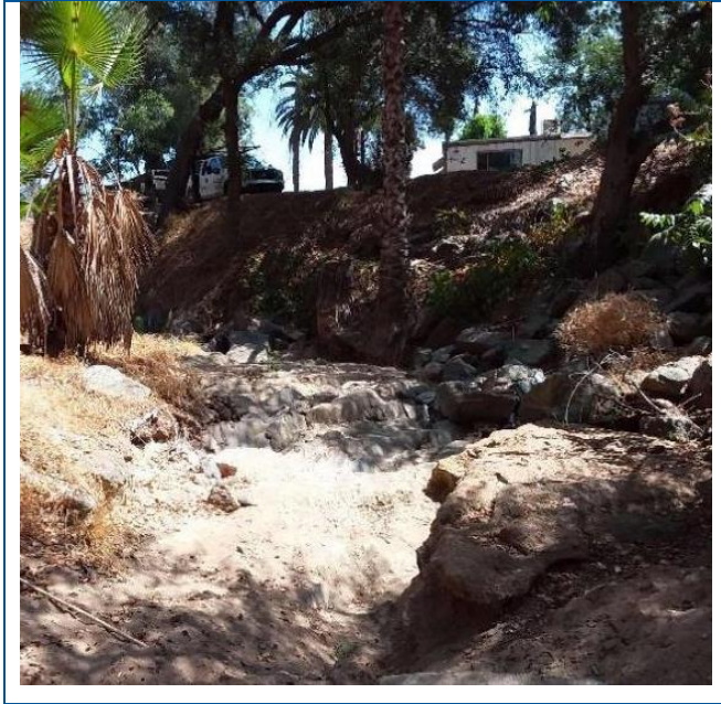
Figure 13 Example of significant stream bank cutting
