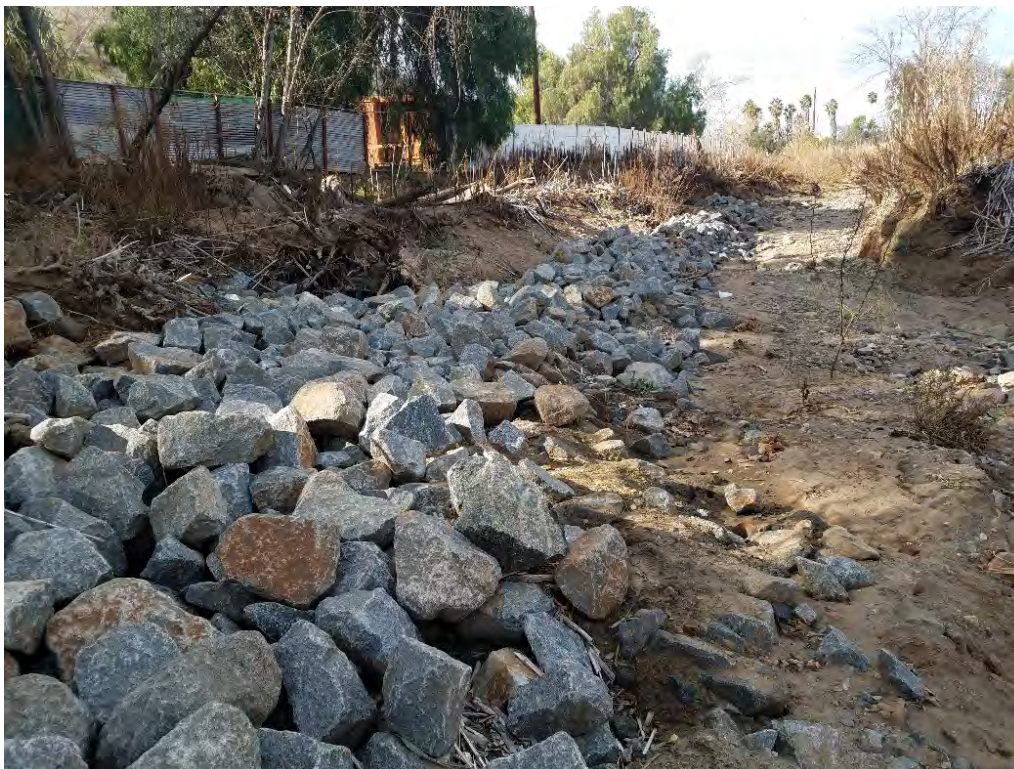
Photograph 1: Riprap Installed within Los Coches Creek. Facing West.
