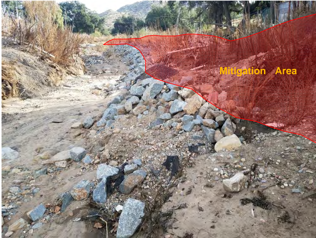
Photograph 2: Mitigation Area 1 along Southern Bank with Installed Riprap. Facing East.
