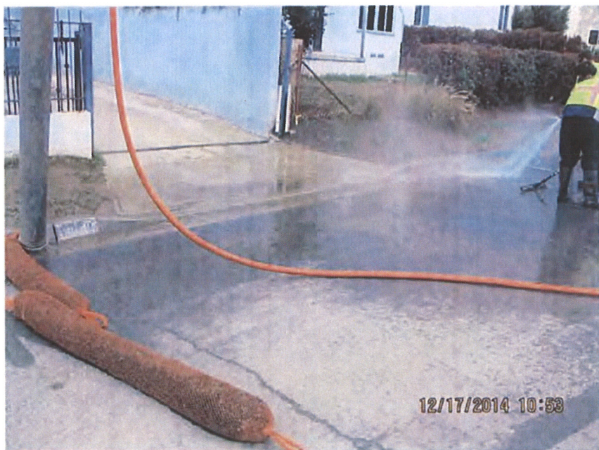
Photo 6. Power washing activity performed by Downstream Services
