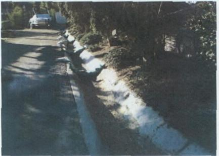
Photo 6: Sediment discharged to MS4 from erosion in previous photo.
