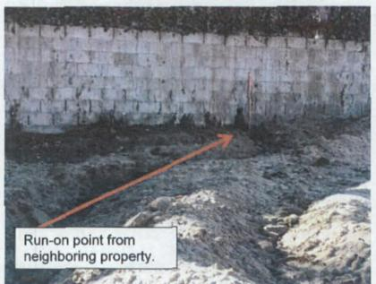
Photo 4: Lack of run-on protection from slope drain from neighboring residence that discharged to dog park area.
