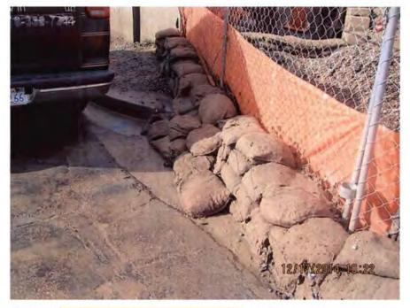
Photo 1. Evidence of sediment discharge at Akins entrance/exit
