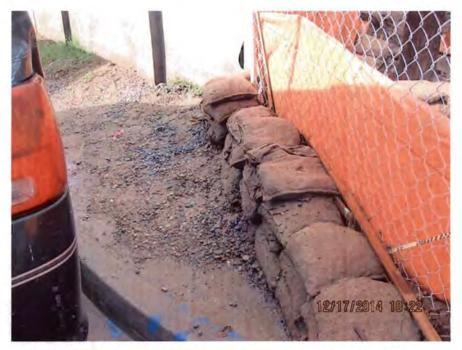
Photo 2. Evidence of sediment discharge at Akins entrance/exit
