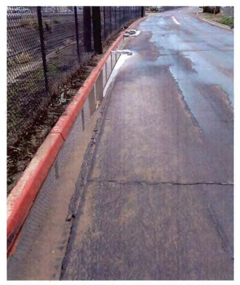
Photo 5. Sediment Accumulation along Akins Avenue, Close to Inlet
