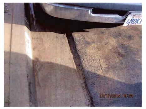
Photo 3. Sediment accumulation along Akins curb gutter, downstream of Akins entrance/exit
