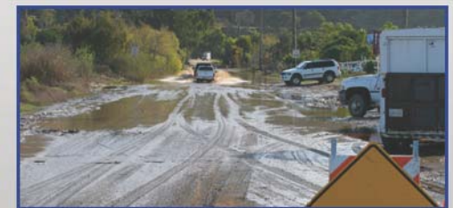
Flooding along Hollister Road in the Valley.
