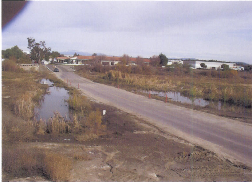
Figure 2. Via Montezuma Road Crossing Murrieta Creek
