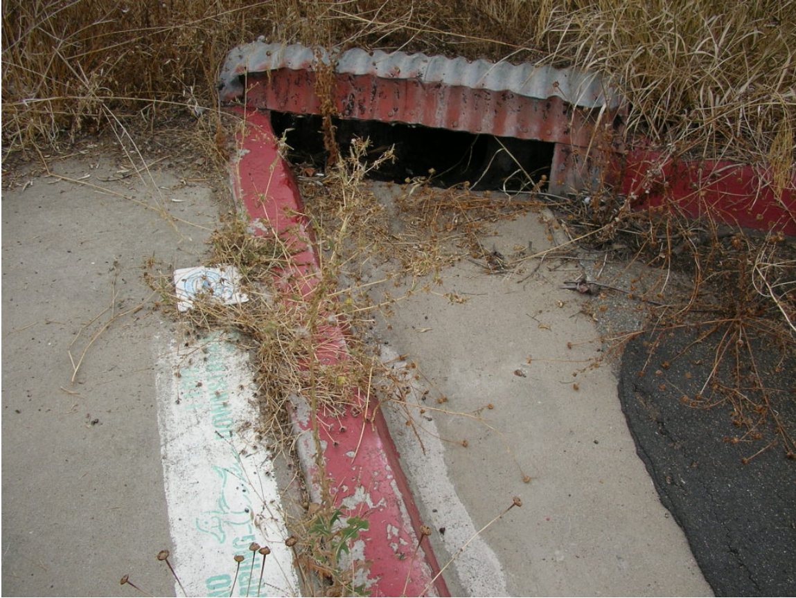
Figure I.4. Roadways land use in Chollas Creek watershed located at the intersection of Quince Street and Chollas Parkway.
