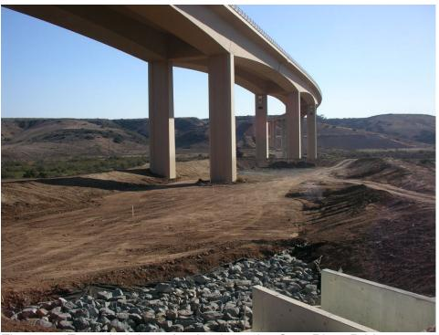
Figure 2. Extended detention basin under Otay River Bridge
