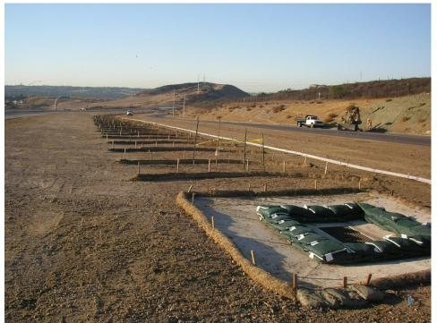
Figure 8. Median bio-swale North of E. H St.
