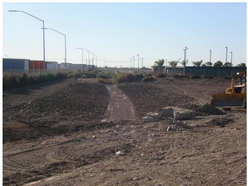
Figure 3. Recently graded bio-swale south of Operations Center building.
