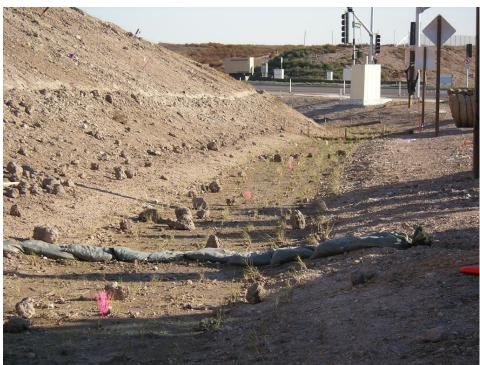
Figure 6. Bio-swale at Birch Rd. (East side)
