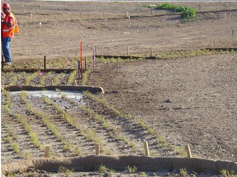
Figure 7. Bio-swale at Birch Rd. (West side)
