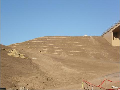
Figure 1. Slope stabilization adjacent to extended detention basin under Otay River Bridge
