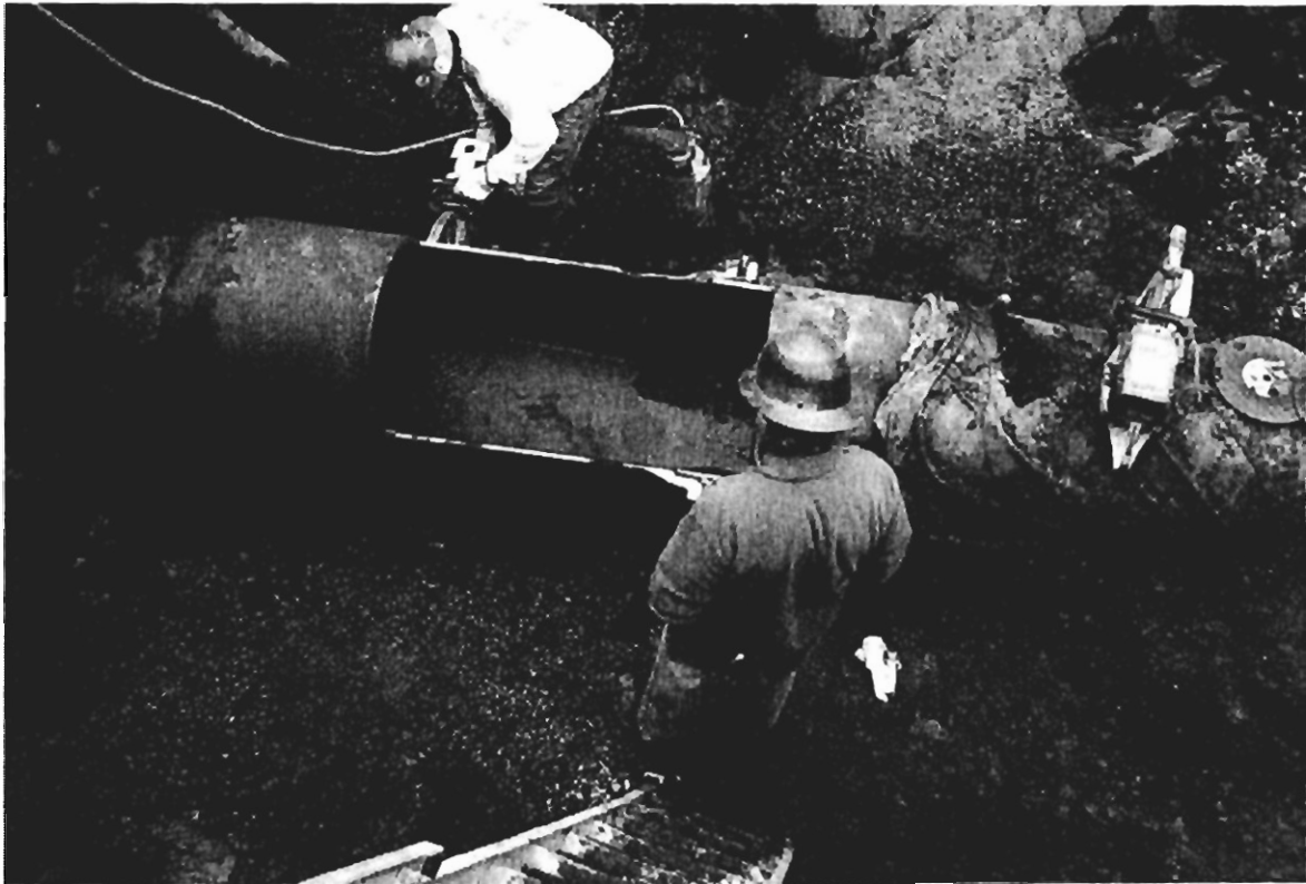
Corroded segment of pipe being removed.
