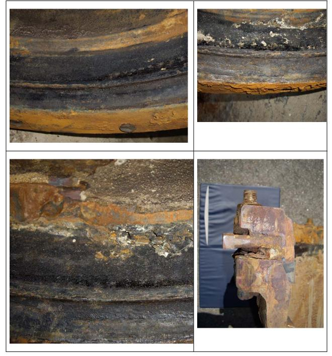
Figure 6 – Four photos showing asphaltic coating and joint condition
