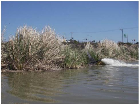
**W43-10: Date:** April 3, 2007 **Time:** 12:06pm. **Photographer:** N. Woodward **Description:** Aeration pump used to increase DO in East Basin **View:** Northeast
