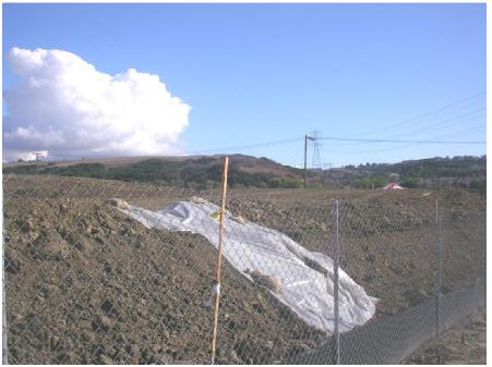
Photo 5 Plastic Spillway For Sediment Trap (Facing Southeast)
