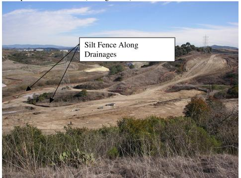
Photo 2 Example of Silt Fence Along Interior Drainages (Facing Northeast)
