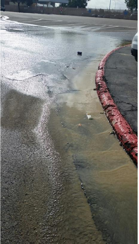
**Photo 5** shows the sediment laden storm water discharged from the site at Anna Avenue and Pacific Coast Highway.
