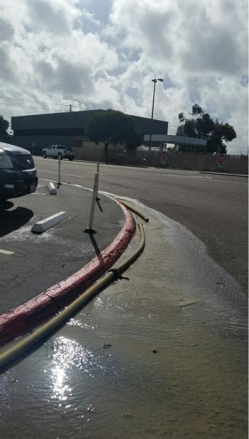
Photo 6 shows the sediment laden storm water discharged from the site at Pacific Coast Highway onto Anna Avenue.
