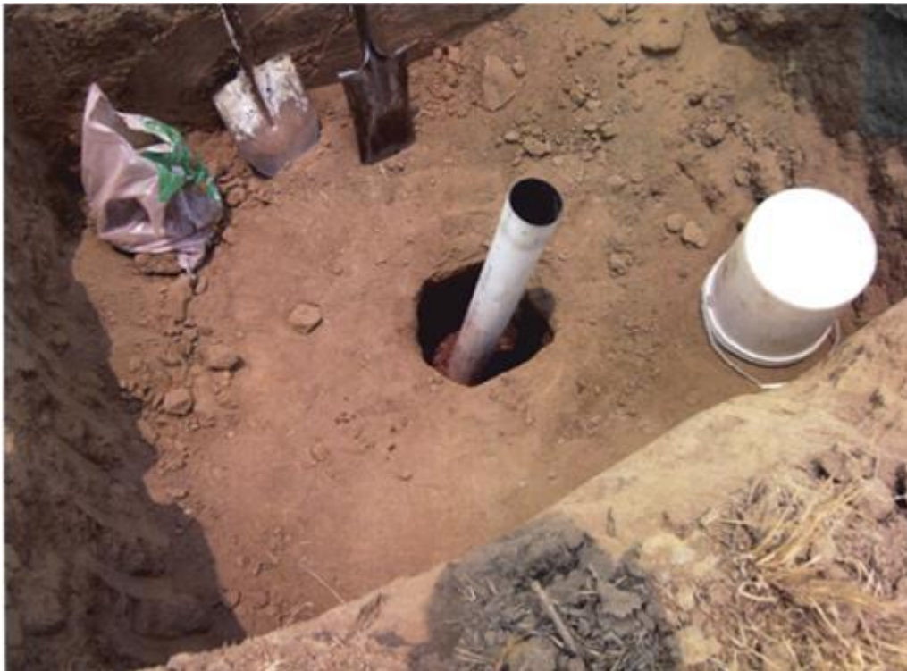
Figure VII.17. Photo of Percolation Test Pit.
