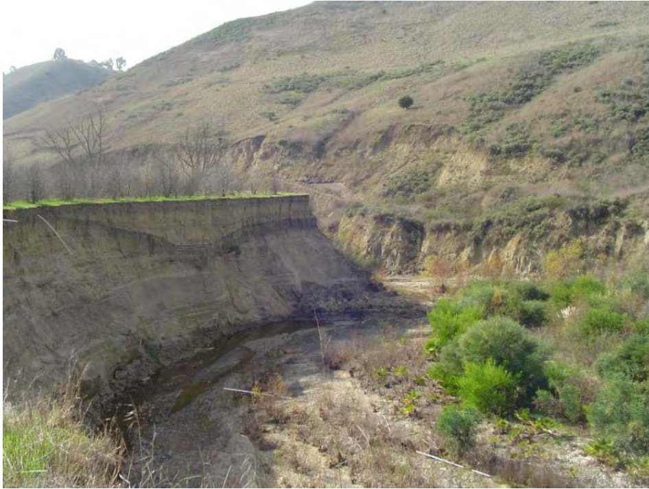
Oso Creek, approximately 1 kilometer (0.7 miles) downstream of a hardened channel
