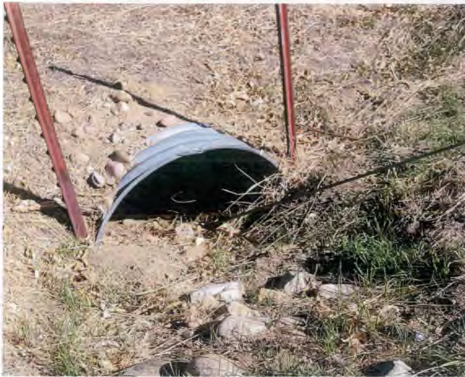
Figure 5-Perimeter Drainage Outlet
