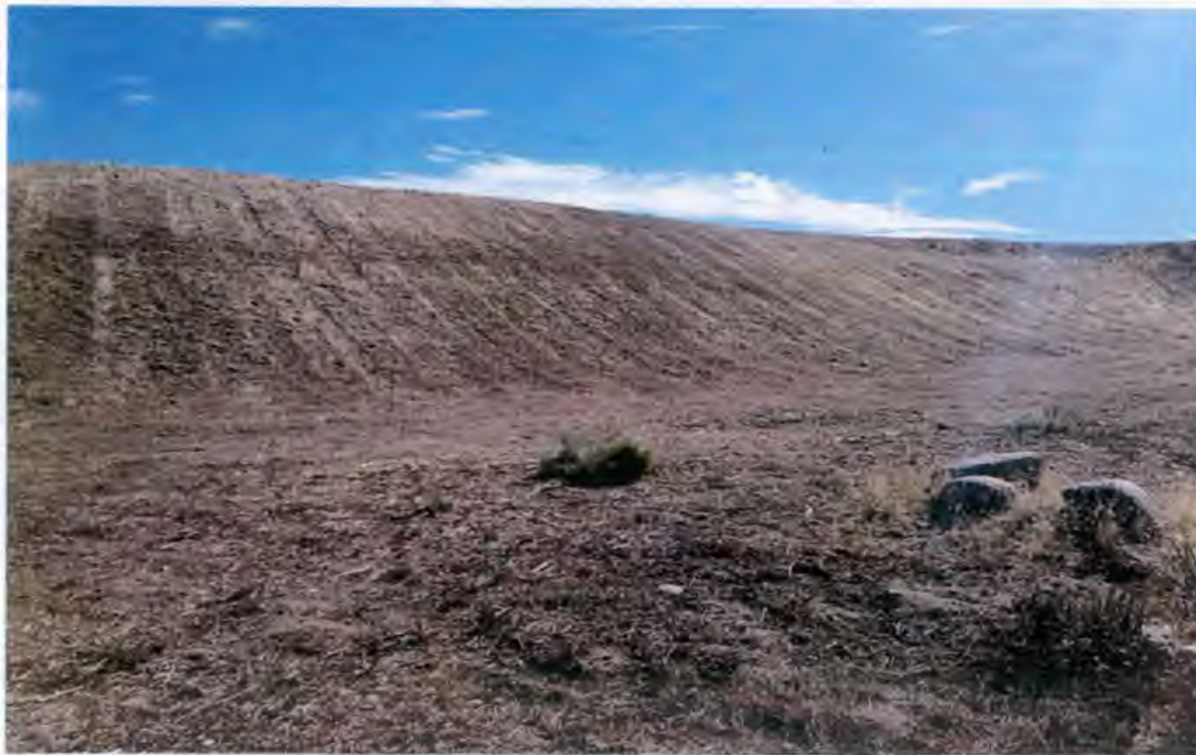
Figure 8- Northwest Face of Landfill
