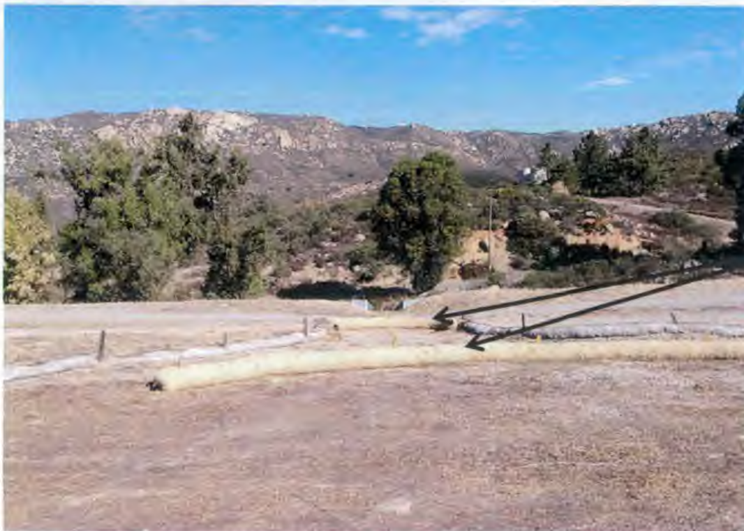
Figure 2- BMPs Implemented in front of Drainage Chute Facing North
