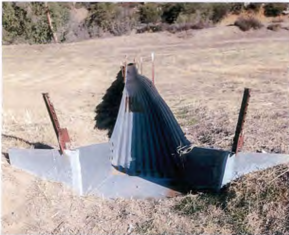
Figure 4- Drainage Chute
