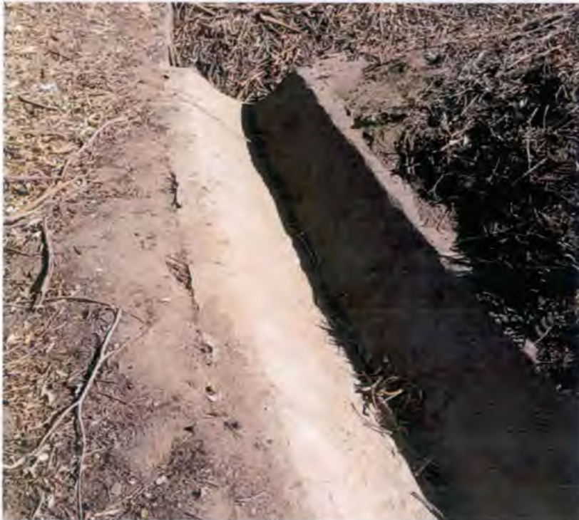
Figure 10- End of Eastern Perimeter Drainage Channel
