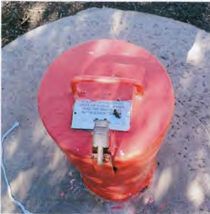
Figure 1- Groundwater Monitoring Well VIGW-3
