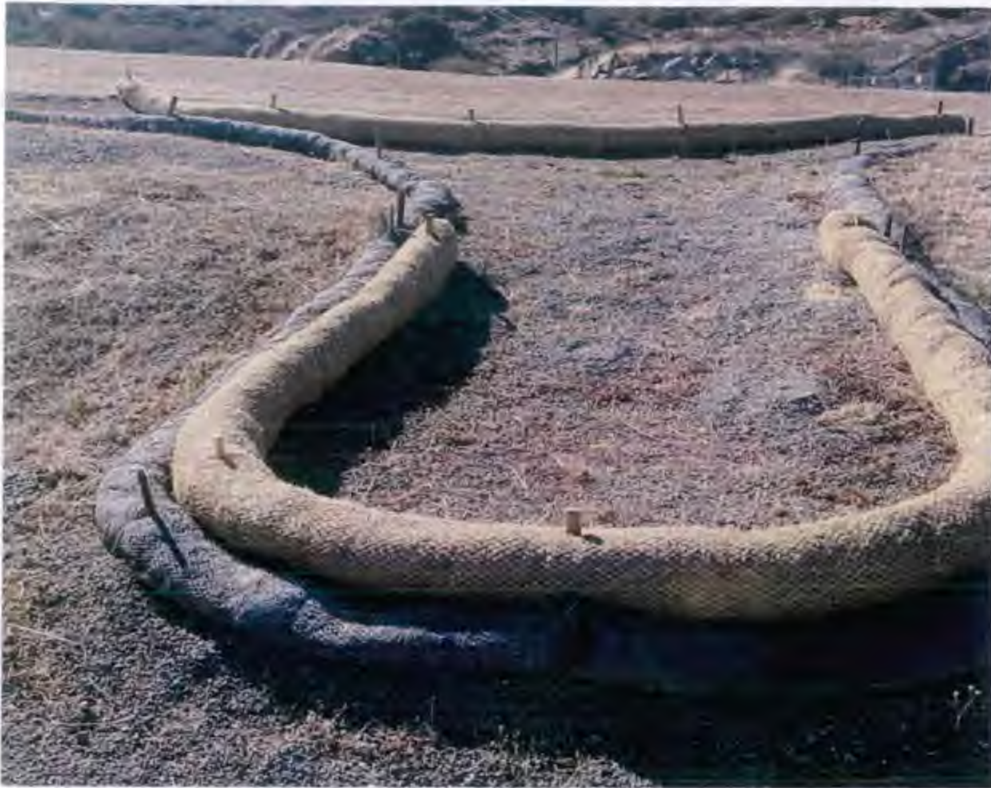
Figure 3- BMPs Installed near Drainage Chute Facing South
