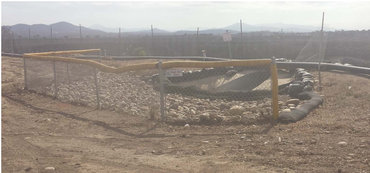
Figure 2: Photo of perimeter drain.
