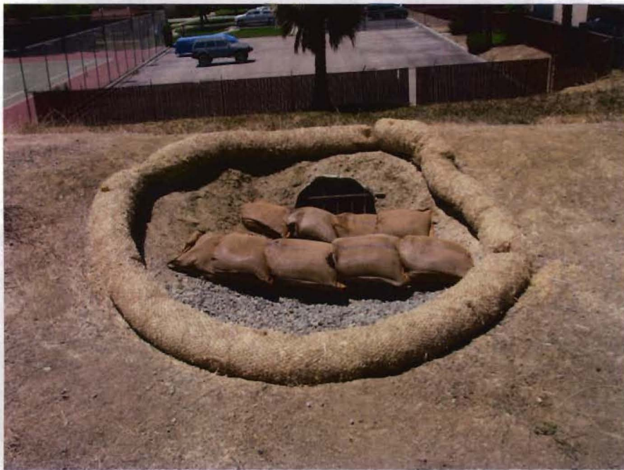
Stormwater BMPs located in the western portion of the Landfill.
