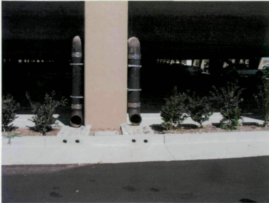
Figure 17. Storm drain piping from roof of parking structure
