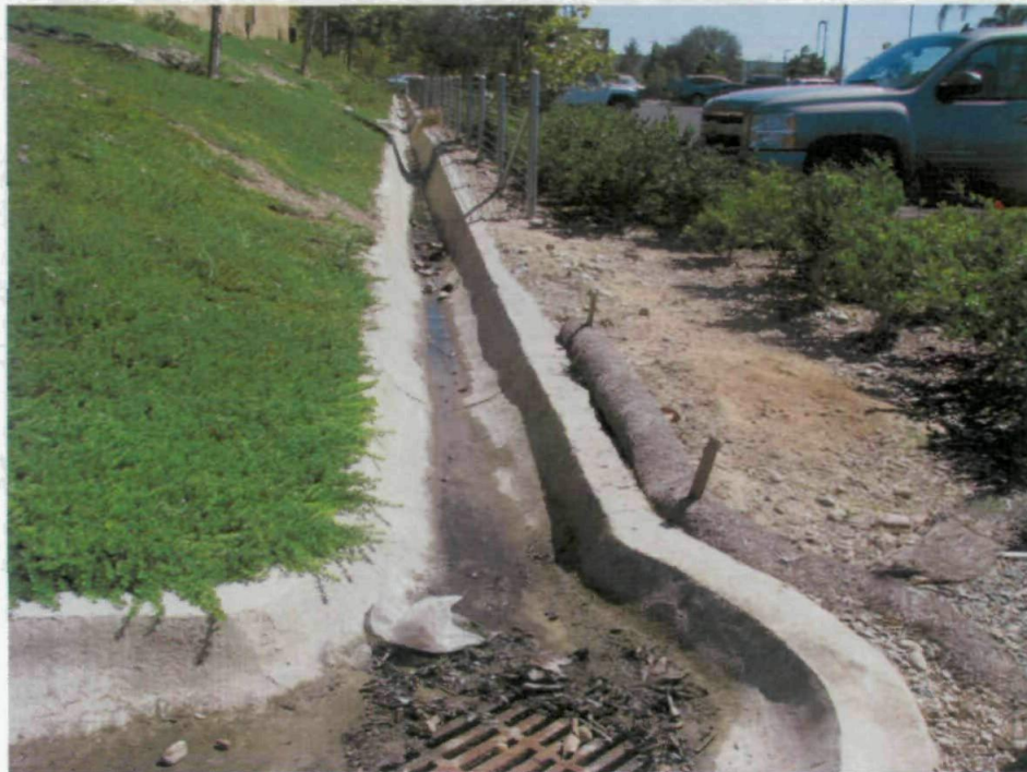
Figure 24. Storm drain system with irrigation runoff
