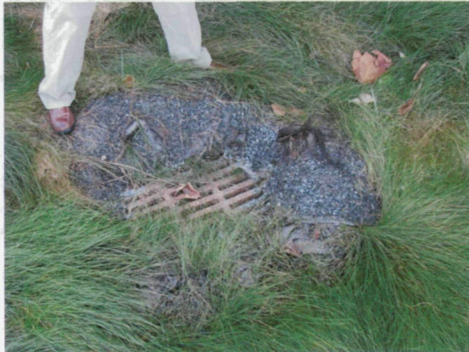
Figure 20. Grass swale outlet
