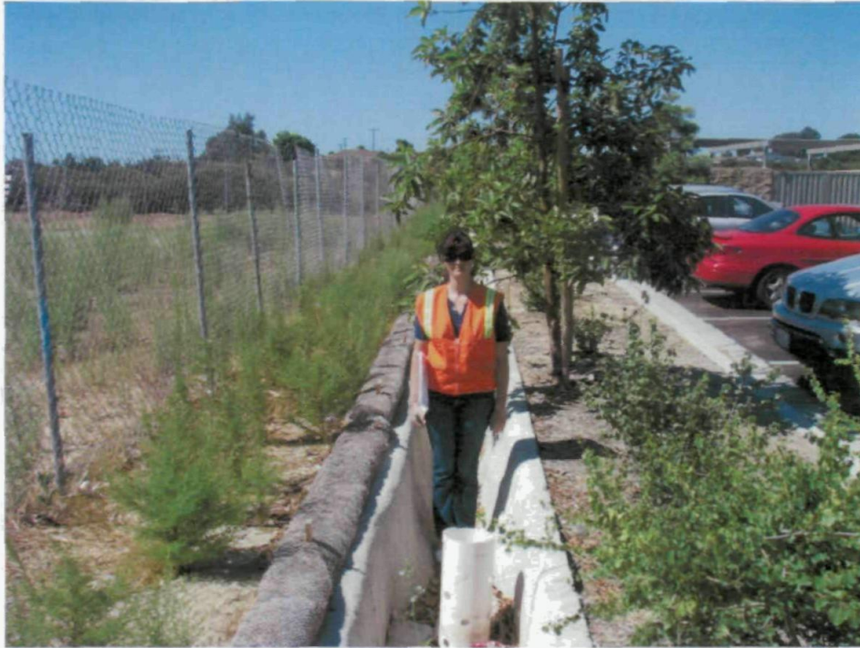
Figure 25. U-ditch on SW side of parking lot
