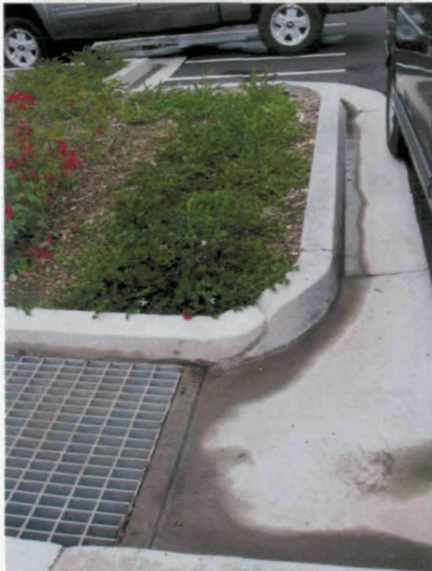
Figure 6. Storm drain receiving runoff from parking lot
