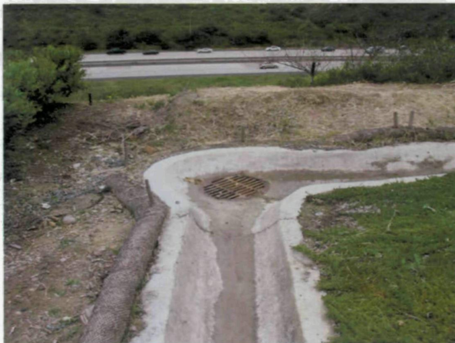
Figure 8. Storm drain receiving runoff from parking lot before leaving site
