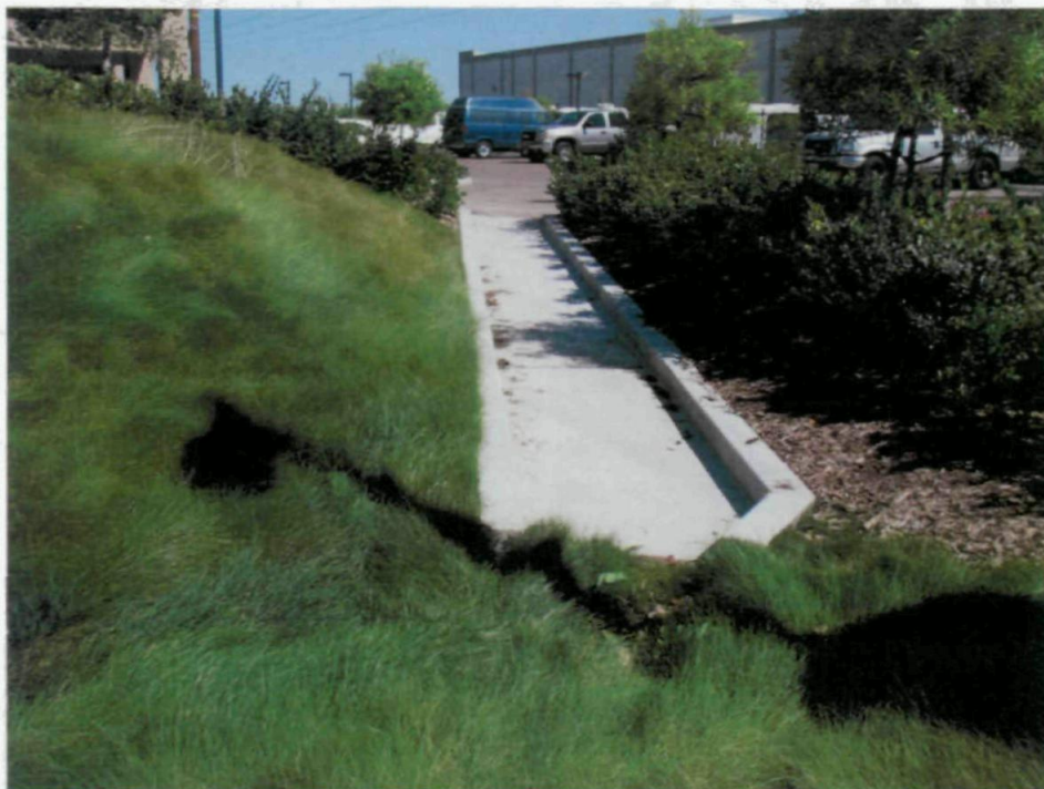
Figure 15. Grass swale inlet
