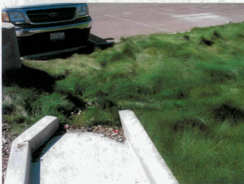
Figure 16. Grass swale inlet
