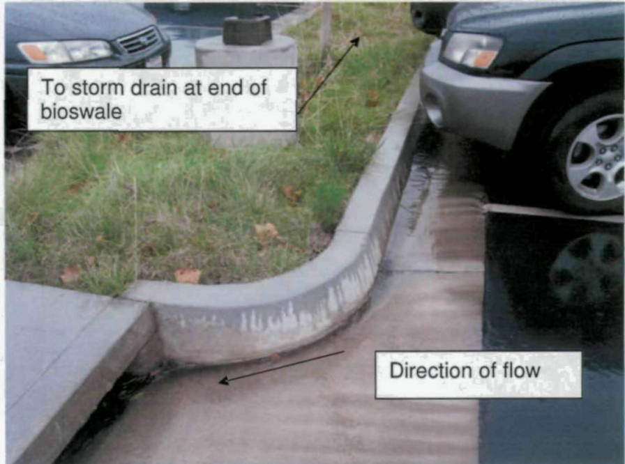
Figure 4. Top of Bioswale 2
