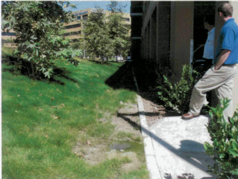
Figure 18. Grass swale inlet (adjacent to parking structure)
