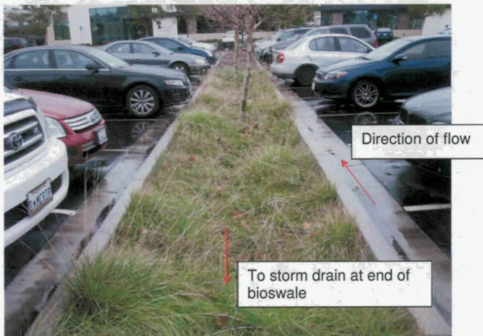
Figure 2. Bioswale 1
