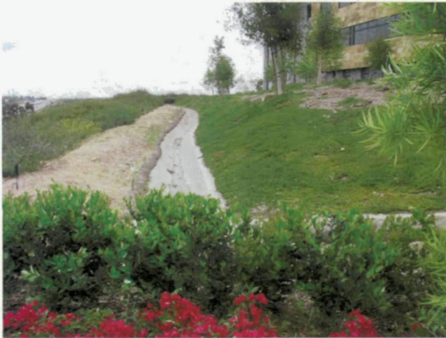
Figure 7. U-ditch receiving runoff from West side of buildings
