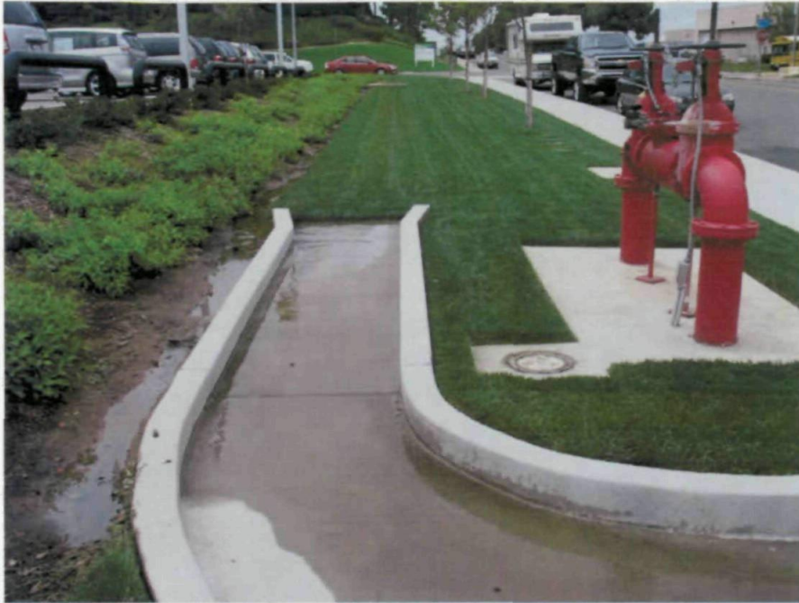
Figure 11. Outlet for Bioswale 1 looking upstream
