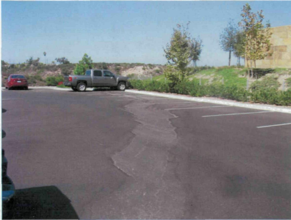
Figure 23. Water stain on asphalt approaches SW corner of lot
