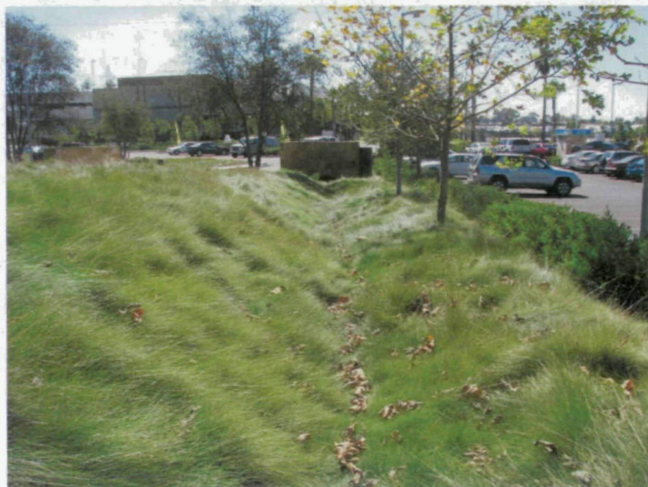
Figure 22. Grass swale on west side looking downstream
