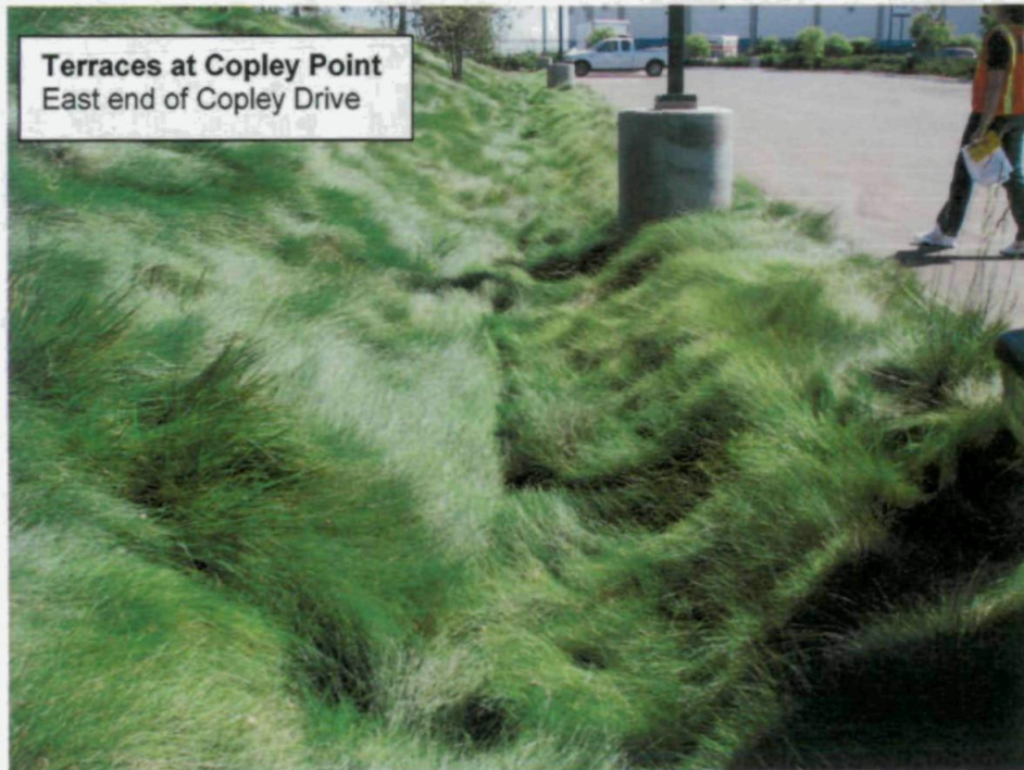
Figure 14. Grass swale at east side looking upstream
