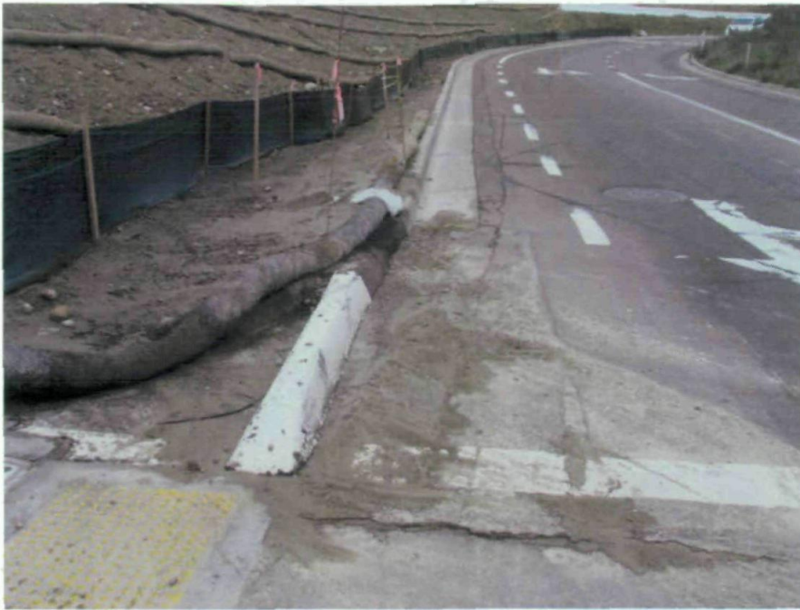
Sediment flow has overwhelmed silt fence and fiber rolls and made its way to conveyance (MS4).
