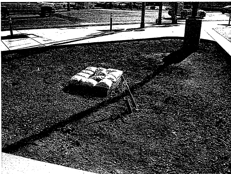
8. Another inlet has been protected. Previously a hole was present in the soil near the inlet that has since been fixed.
