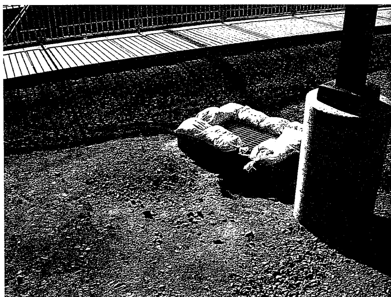
9. Another inlet that has been protected. This inlet does have a hole in the soil near the inlet suggesting that storm water bypasses the inlet and drains through this hole.
