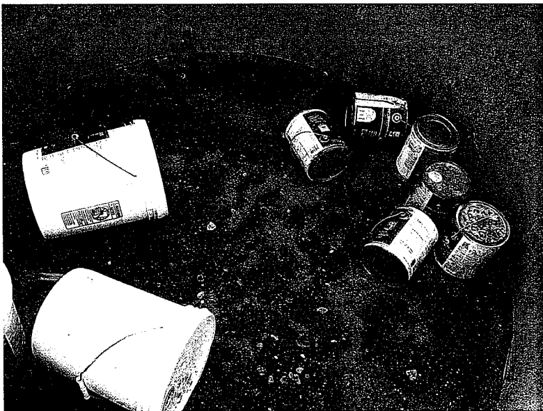
11. At the north west corner of the Escondido Transit Center, large concrete pipe sections were standing on end. Inside one of these pipe sections was stored paint and other construction materials without proper cover or containment to prevent contamination of potential storm water contact.
