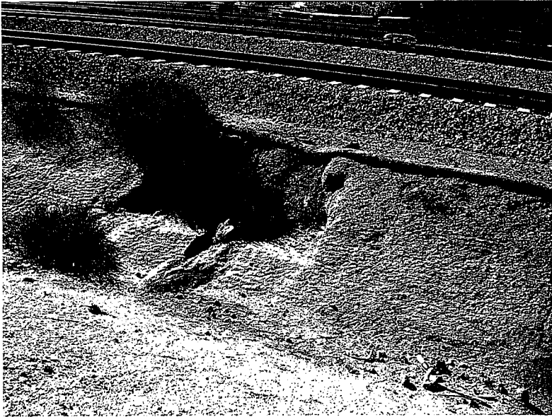
4. An erosion gully is present on the bank of the unstabilized channel.
