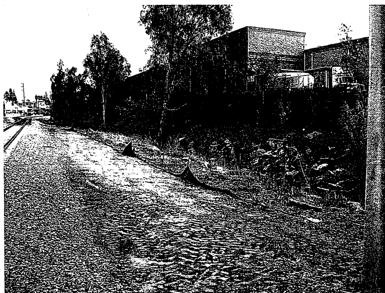
12. At the west end of the Escondido Avenue Center and south of the tracks near the bridge over Escondido Creek, an old silt fence has not been maintained and may become a potential trash pollutant in the nearby channel.
