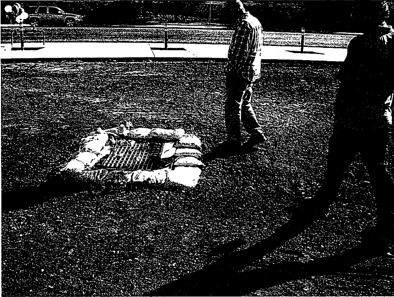
7. Storm drain inlet is protected.
