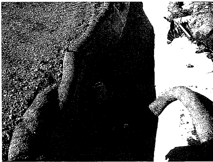
11. Sediment accumulation and fiber roll in need of maintenance.
