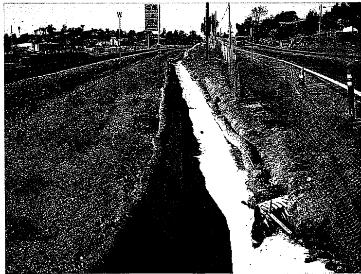
12. Concrete-lined ditch leading to culvert inlet shown in Photo 11. More accumulated sediment.
