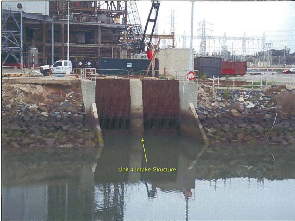
Figure 3. Unit 4 Intake Structure (32.613792, -117.096773)
