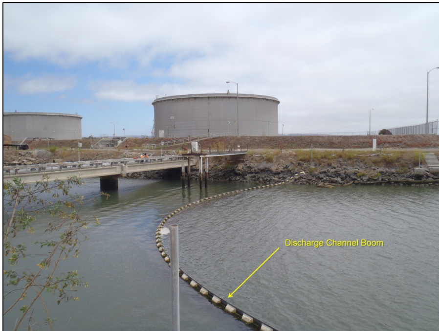
Figure 10. Floating boom at the mouth of the discharge channel (32.613408, -117.098018)
