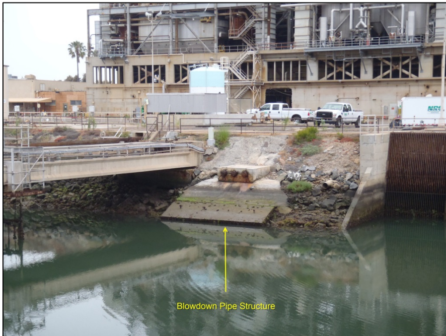
Figure 6. Blowdown pipe structure in the intake channel (32.613939, -117.097148)
