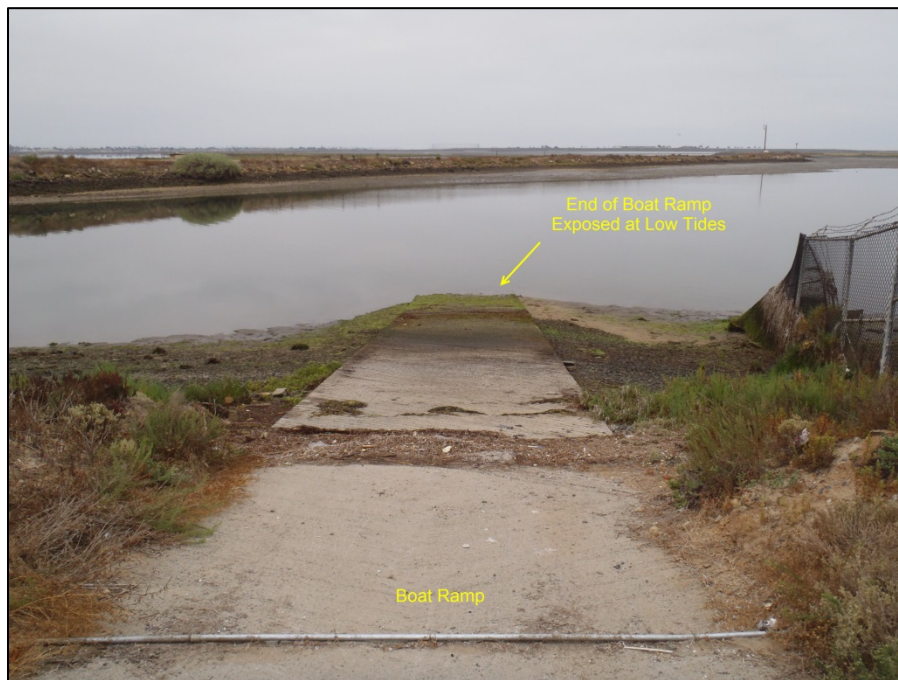
Figure 8. Concrete Boat Ramp in San Diego Bay near the Intake Channel (32.614671, -117.098157)
