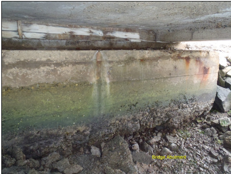
Figure 4. Representative bridge abutment (32.613982, -117.097190)
