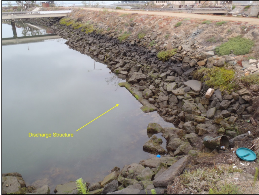
Figure 11. Representative discharge structure in the discharge channel
