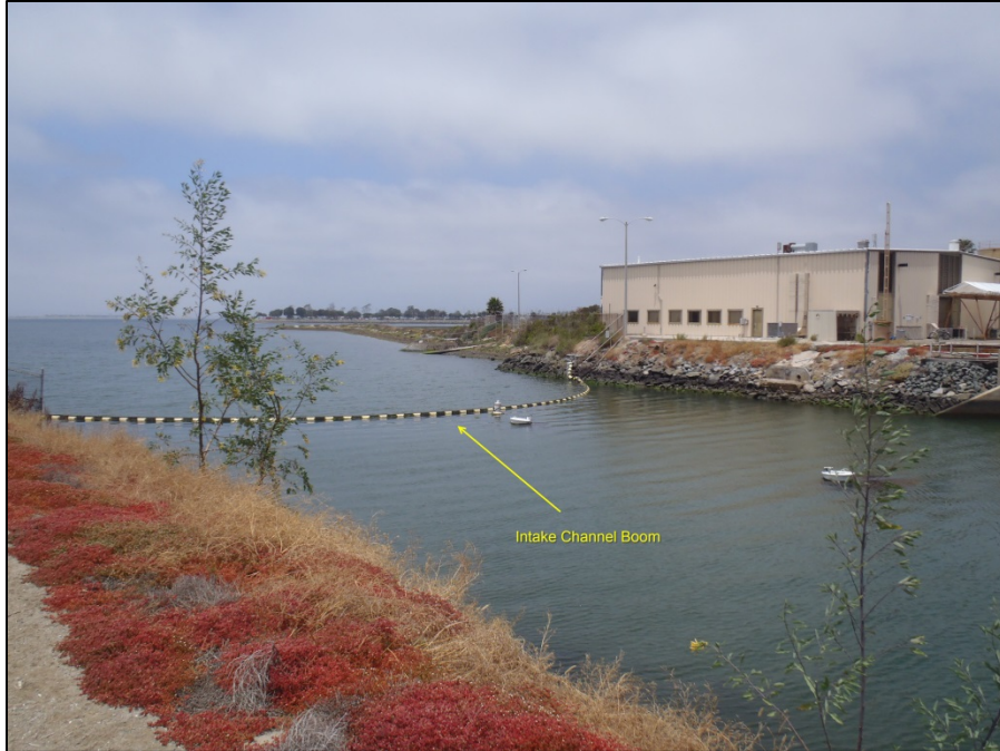
Figure 9. Floating boom at the mouth of the intake channel (32.614111, -117.097950)
