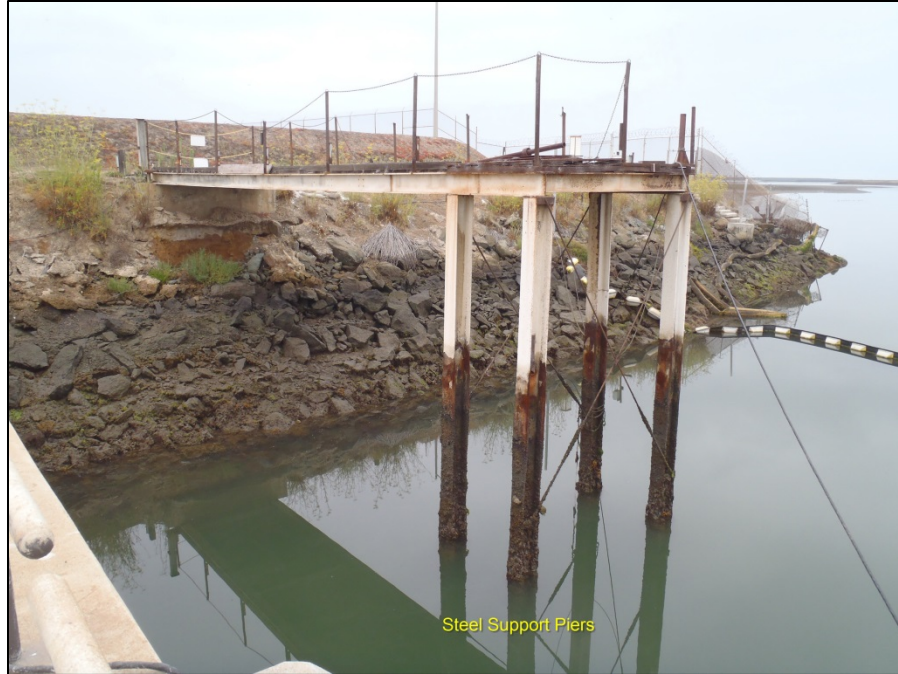
Figure 7. Steel Pier Supports (32.613275, -117.097720)
