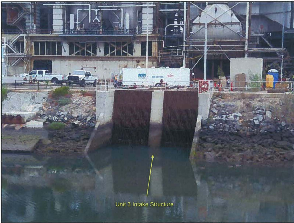
Figure 2. Unit 3 Intake Structure (32.613917, -117.097018)
