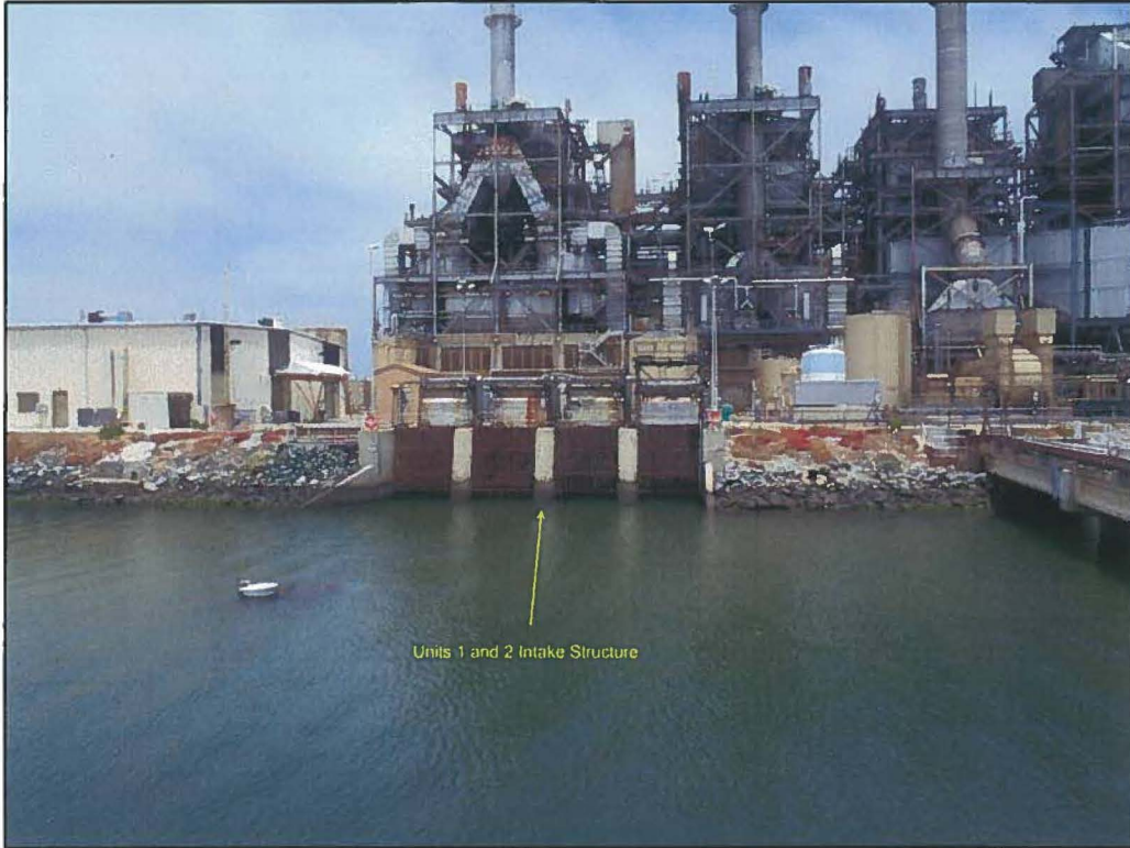
Figure 1. Units 1 & 2 Intake Structure (32.614110, -117.097412)
