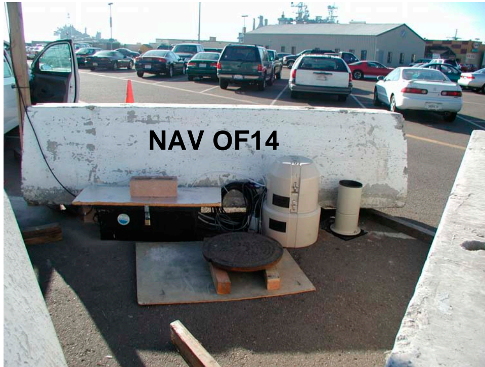
Figure 9. Naval Station San Diego storm water monitoring location for outfall 14. The site was located in a parking lot about 650 feet from the discharge point through the quay wall. The barriers were provided by the base to provide a secure monitoring area.
