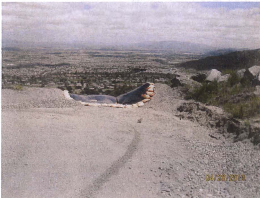
Photo 14. Nunez pad drainage toward temporary Visqueen-lined outlet.
