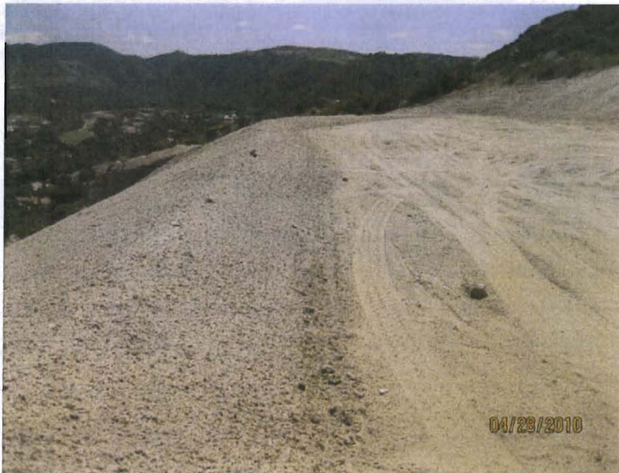
Photo 19. Bonded fiber matrix protection of slope descending from pad 7
