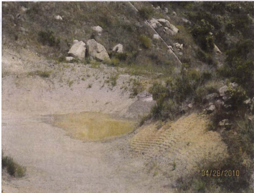
Photo 6. Completed Upper basin looking down from above.
