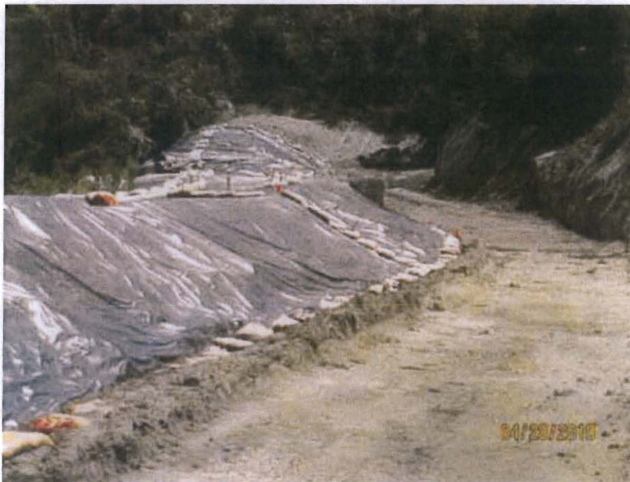
Photo 2. Completed Lower basin. Graded areas to be planted with native vegetation
