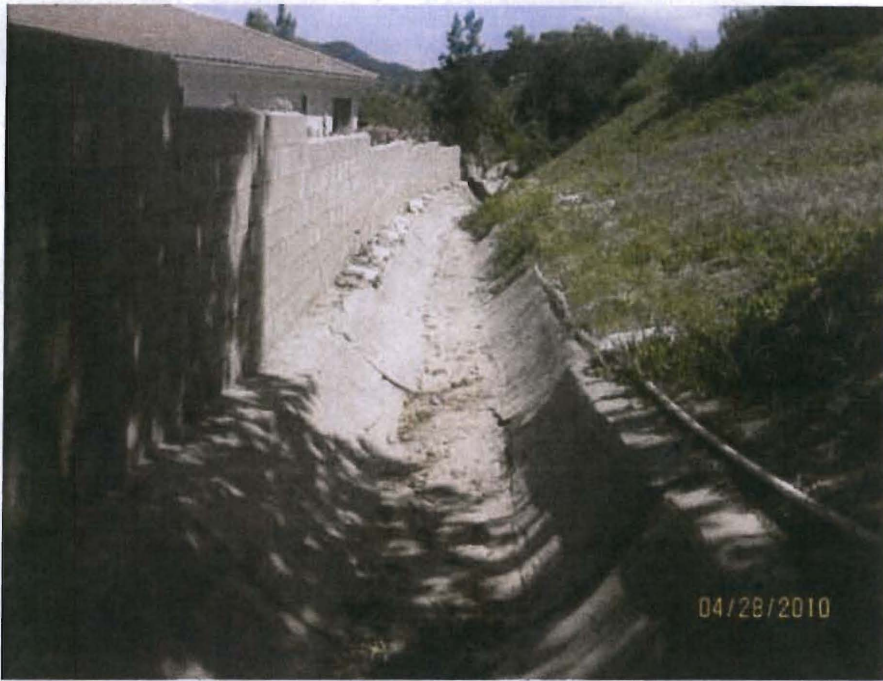
Photo 1. View of Paved Drainage Swale behind 22408 Montes Court
