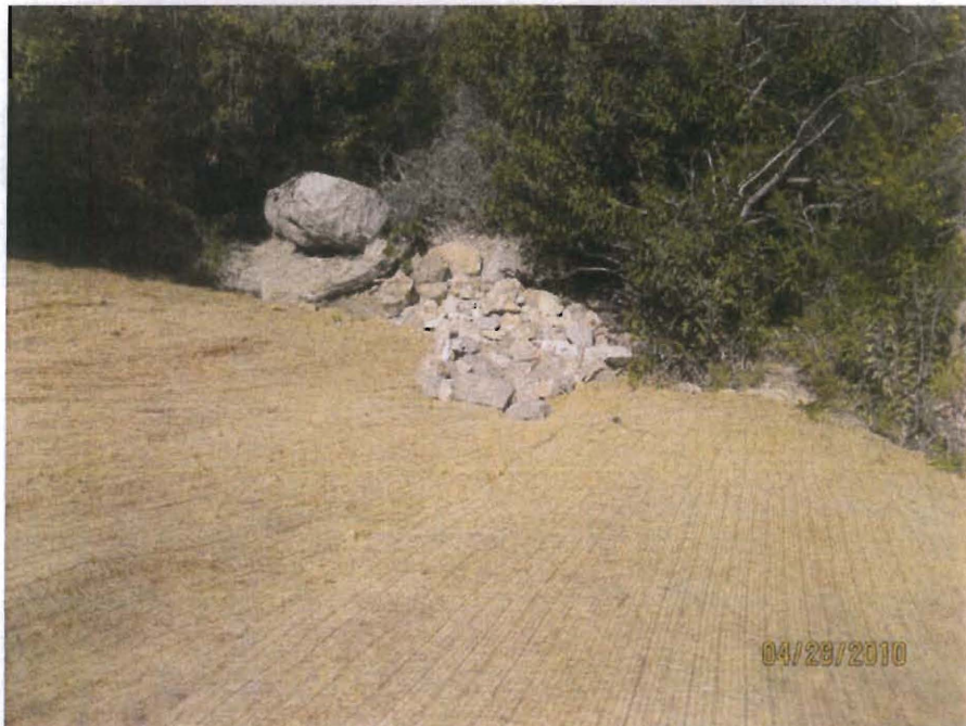
Photo 8. Looking downstream at the outlet and rip-rap below the Entrance Basin. Note jute netting on slope and undisturbed canyon below
