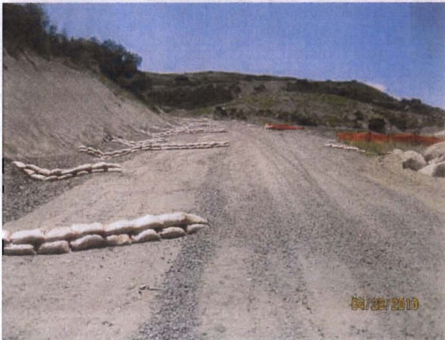
Photo 4. Gravel Chevrons and slope protection, Via Vista Grande.
