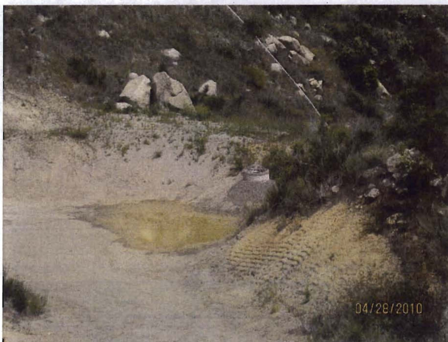
Photo 6. Completed Upper basin looking down from above.
