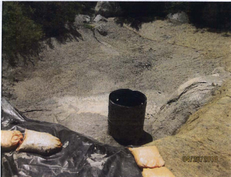
Photo 7. Riser pipe in completed Entrance basin
