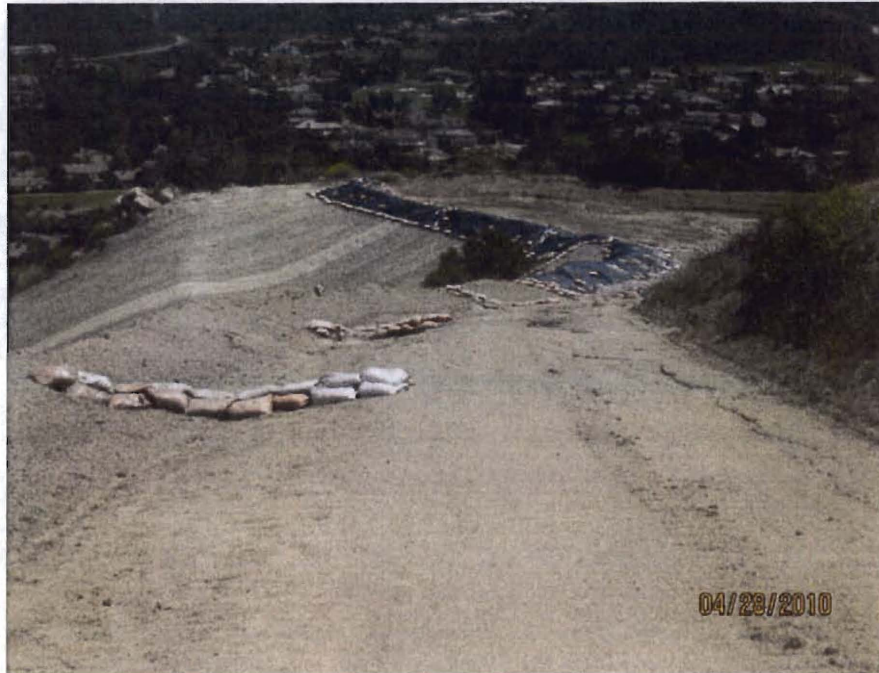
Photo 21. Looking down driveway to pad 8
