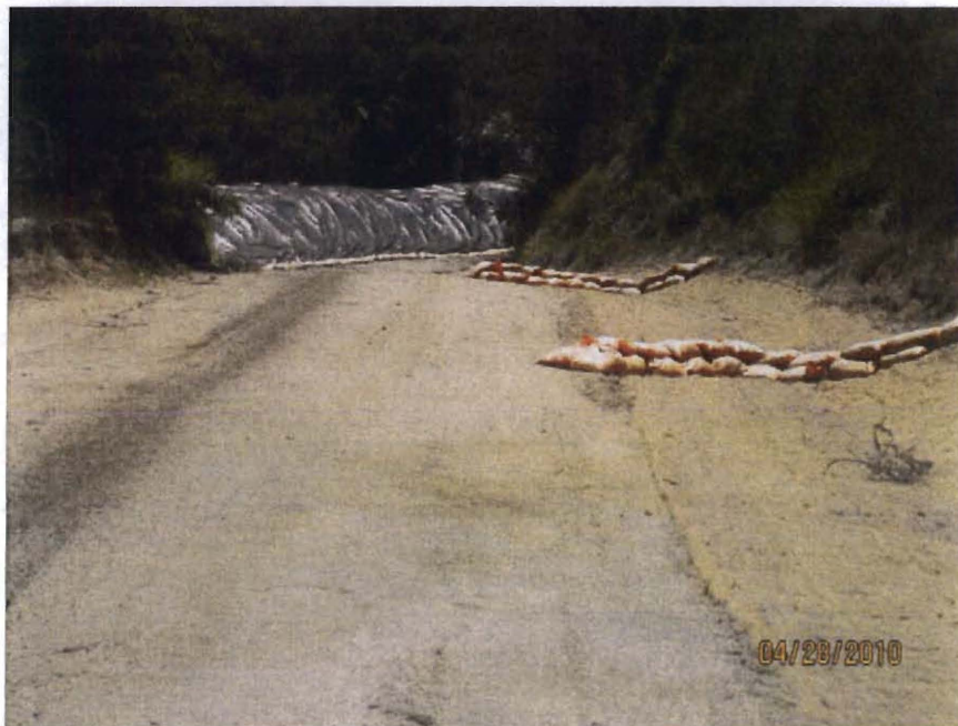
Photo 16. Looking down Cheeks Road to Lower Basin. Note erosion control mat and sandbags on inside of road
