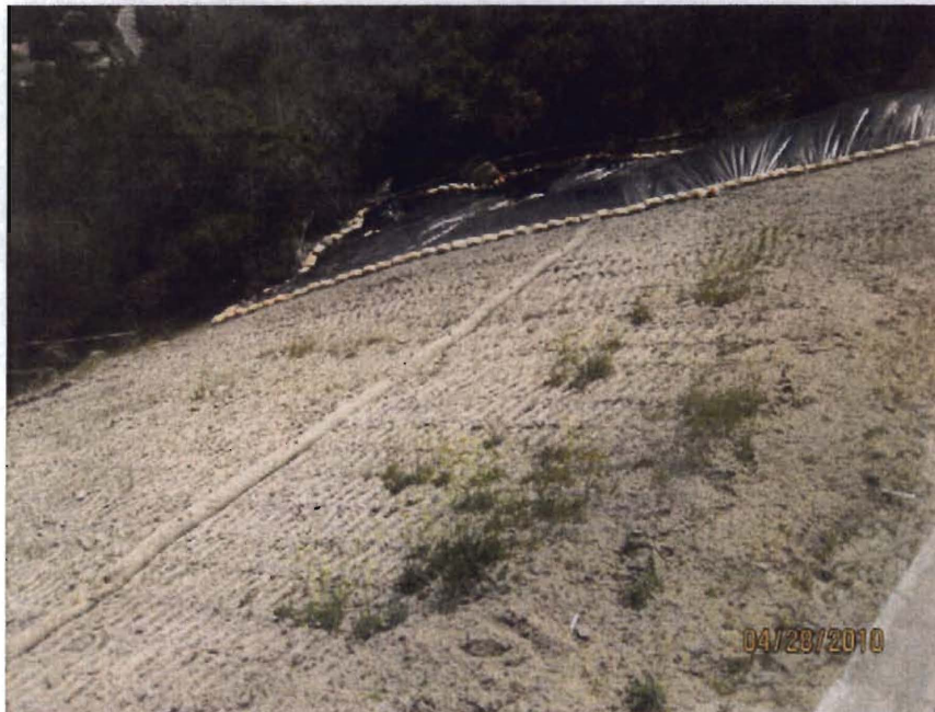
Photo 18. Slope descending from Ragsdale pad. Note temporary down-drain with Visqueen protection.
