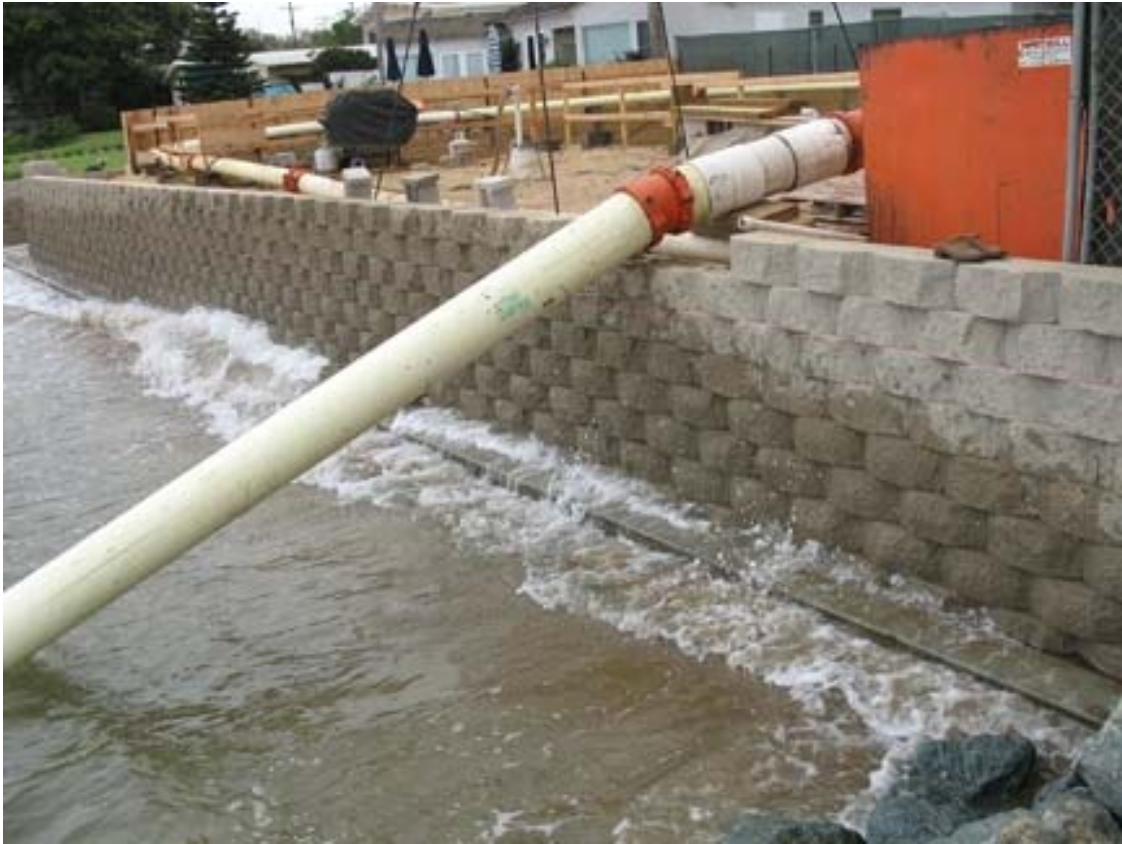
View to the south of 501 First St. (Oct. 9, 2006)
