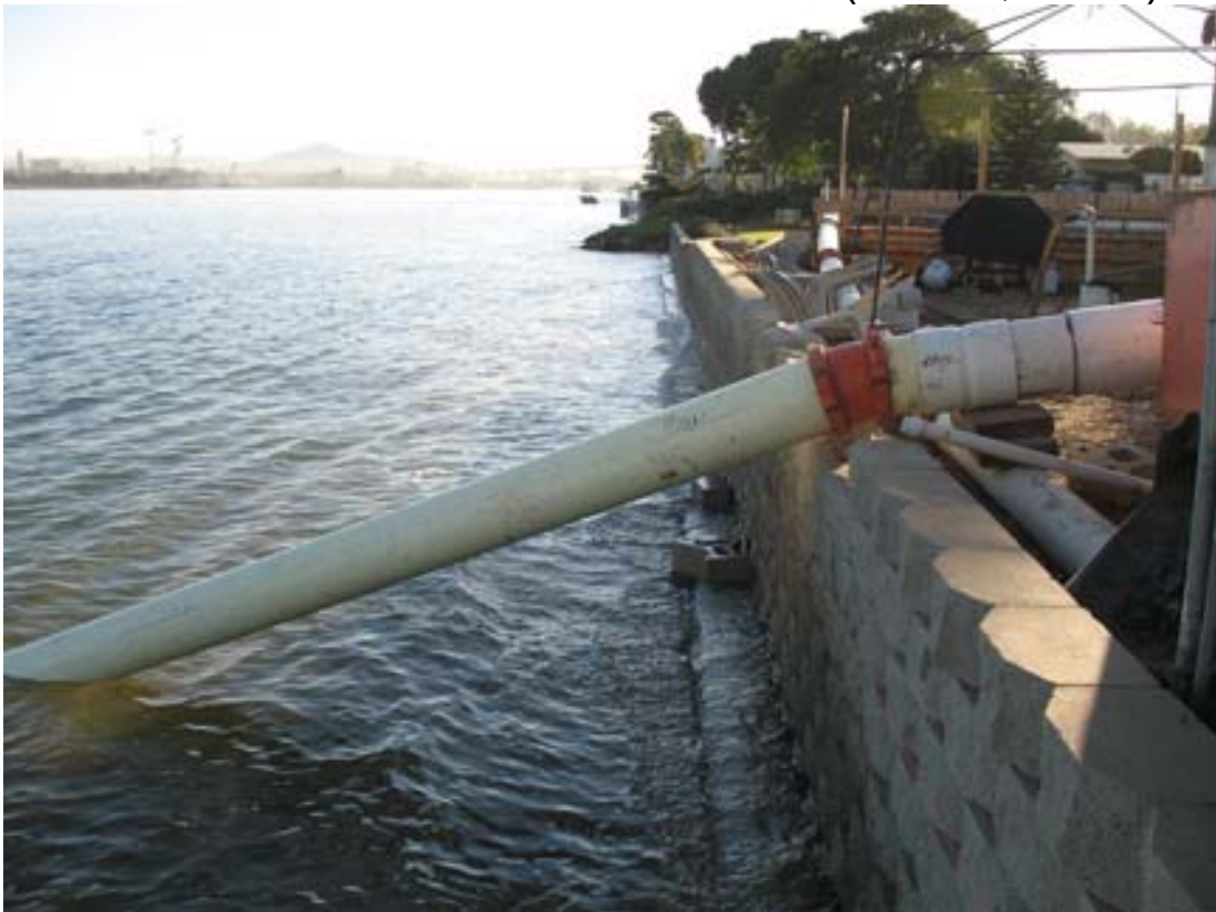
View to the southeast of 501 & 505 First St. (Dec. 4, 2006)
