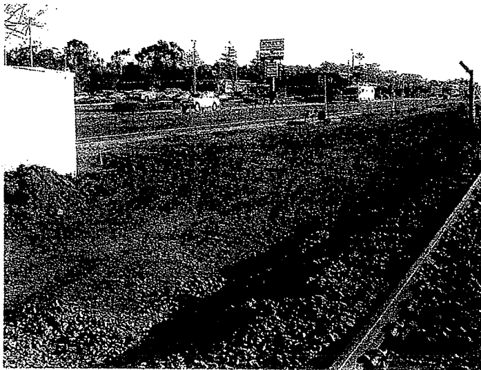
Photo 2 Repair to photo 2 in the NOV. Fiber rolls in place to provide sediment control.
