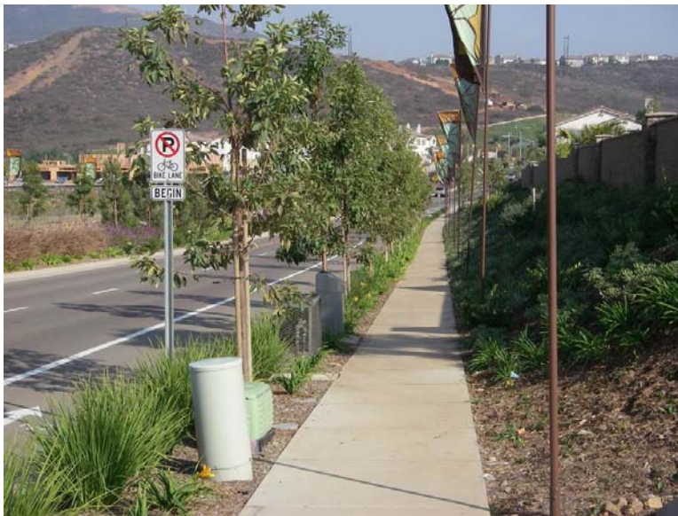
Figure D-7. Vegetative Strip in Residential Area, San Elijo Hills, Carlsbad Watershed
