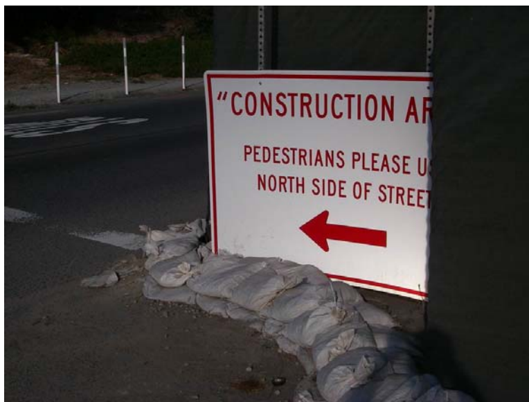
Figure D- 4. Use of Sandbags upstream of Moonlight State Beach, Encinitas Blvd., Carlsbad Watershed.
