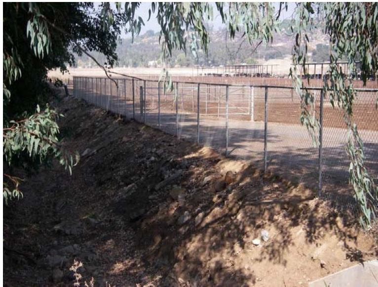
Figure D-1. Animal Exclusion Device at Konyn Dairy, Valley Center Road, San Dieguito Watershed.
