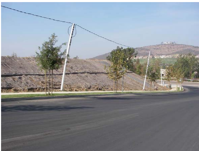
Figure D-3. Use of Netting and Fiber Rolls at San Elijo Hills Construction Site, Northstar Way, Carlsbad Watershed.
