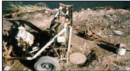
Figure 156: Sewer cleanout underway at Av. Reforma (Nov 1994)
