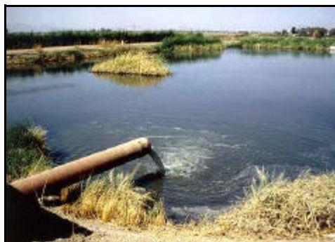
Figure 145: Influent to Gonzalez-Ortega treatment facility (Aug 1994)
