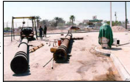
Figure 176: Work underway to correct problems at Pumping Plant No. 3 (formerly PP1A) (Aug 1995)
