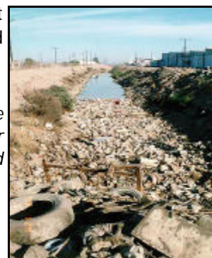
Figure 183: Mexicali Drain at Highway 2 (Jan 1995)
