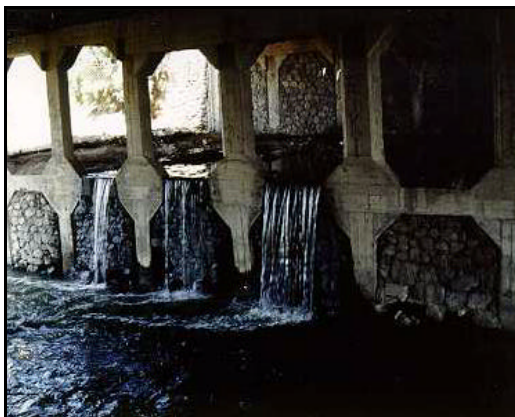
Figure 142: Bypass of raw sewage at Av. Reforma crossing from east bank (Aug 1994)
