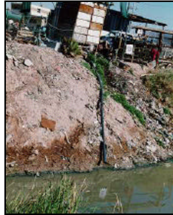
Figure 161: Outhouse discharging to Mexicali Drain (Feb 1995)
