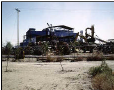
Figure 151: Siderurgica California, a steel recycling plant (Oct 1994)
