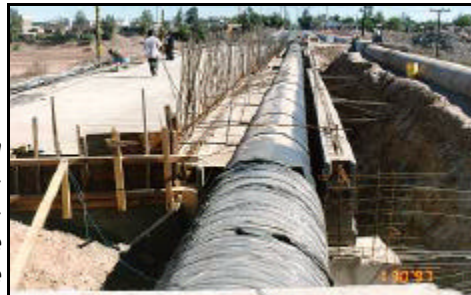
Figure 188: Replacement of concrete pipe with steel pipe on the South Collector (Jan 1997)
