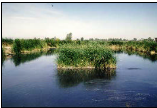
Figure 168: Gonzalez-Ortega sewage treatment lagoons (Apr 1995)
