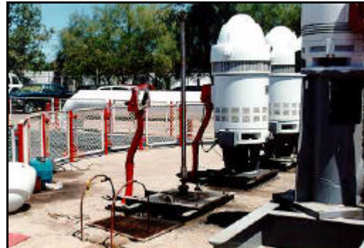
Figure 181: Repairs underway at Pumping Plant No. 1 (Apr 1995)
