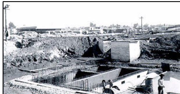
Figure 2: Construction of Pumping Plant No. 2 underway (Dec 1964)
