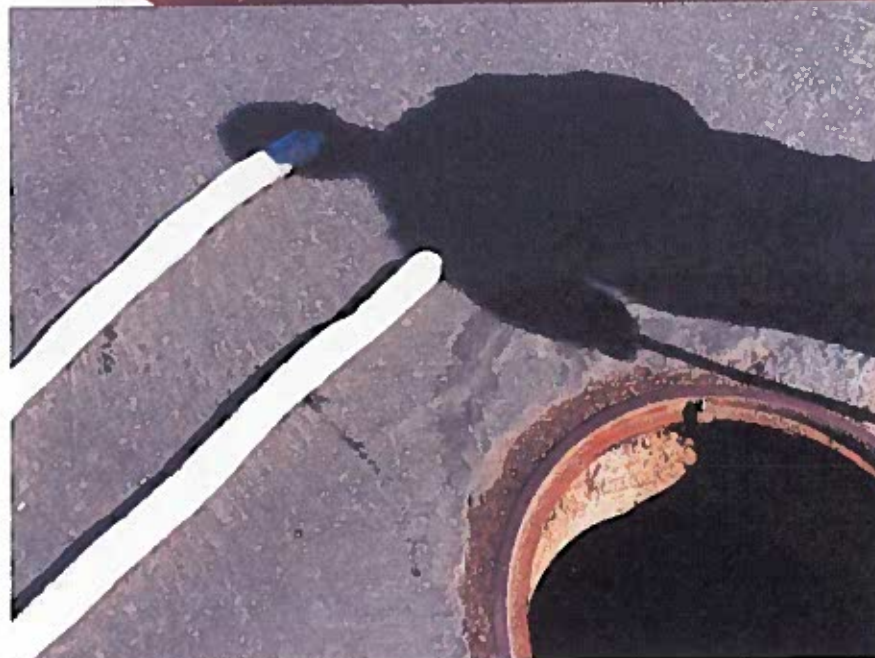
Absorbent boom after placement in storm drain pipe upstream from Ski Run Marina, no oily material present
