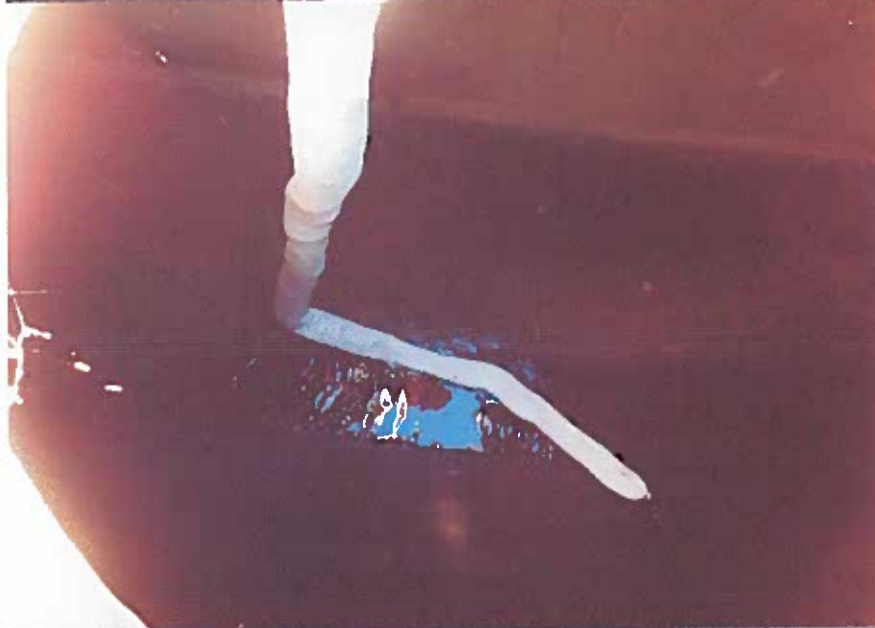
Absorbent boom in upstream storm drain
